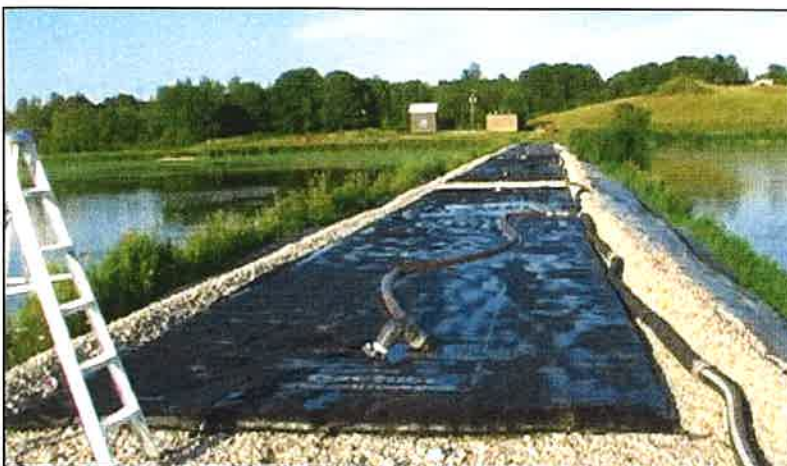
In August 2009, Six Geotube® units were used to dewater and contain sludge pumped from one of the three sewage lagoons operated by The Municipality of Arran-Elderslie.
