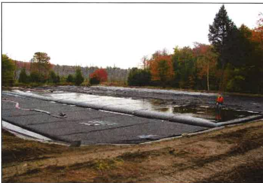
Geotube® units were deployed atop a dewatering cell constructed of an impermeable geo-membrane material designed to collect the filtrate pouring from the bags. Collected filtrate was discharged to the lagoon.
