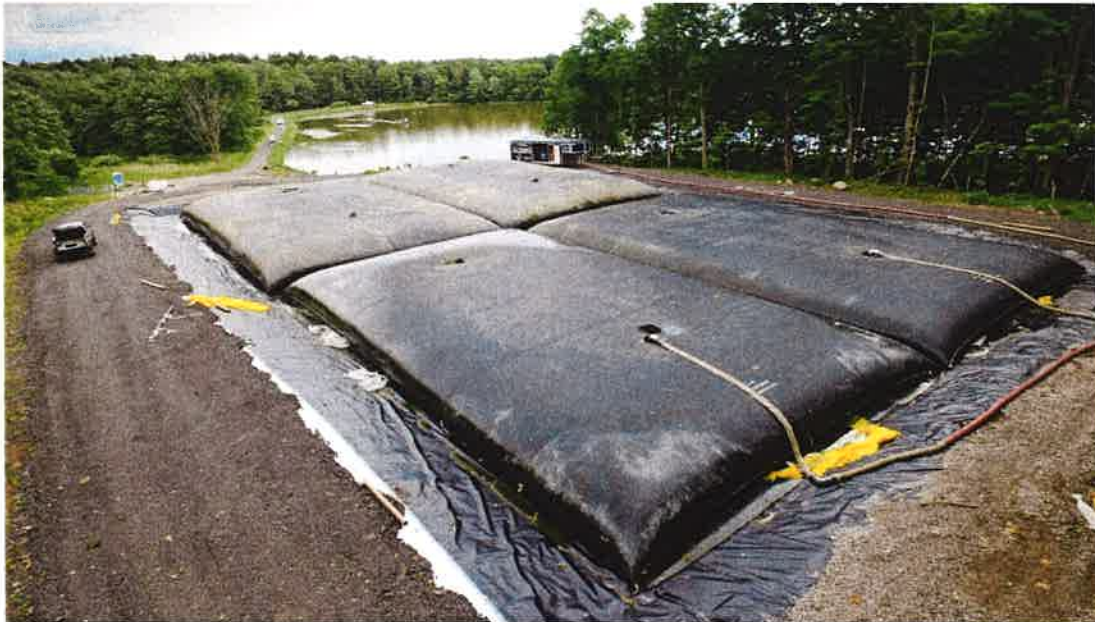
Figure 4. Geotube® dewatering cell constructed using impermeable liner and non-woven geotextile.
