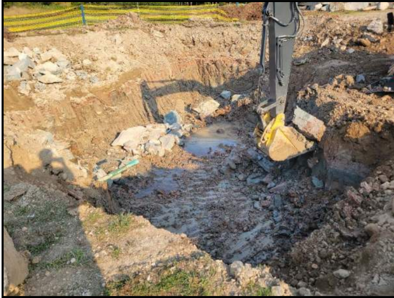
Photo 1 – View of the remedial excavation activities.
