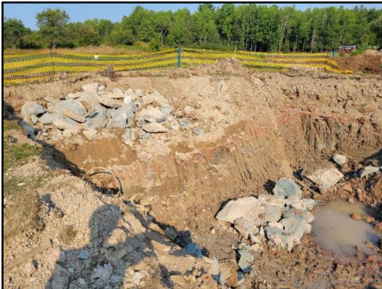
Photo 2 – View of the northwest excavation wall.
