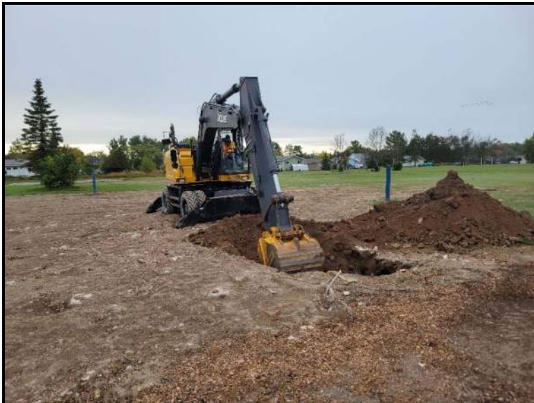
Photo 4 – View of the beginning of remedial excavation activities.
