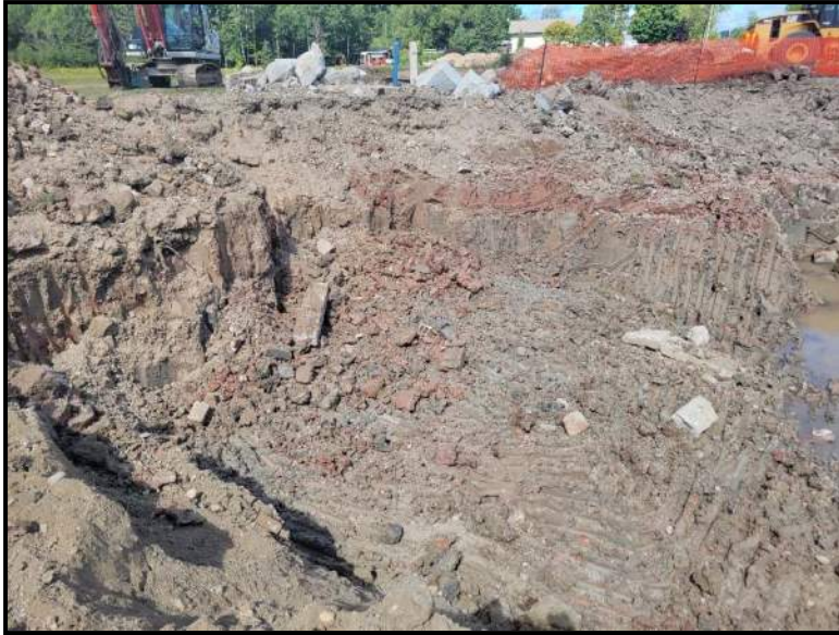
Photo 3 – View of the remedial excavation, looking northwest.
