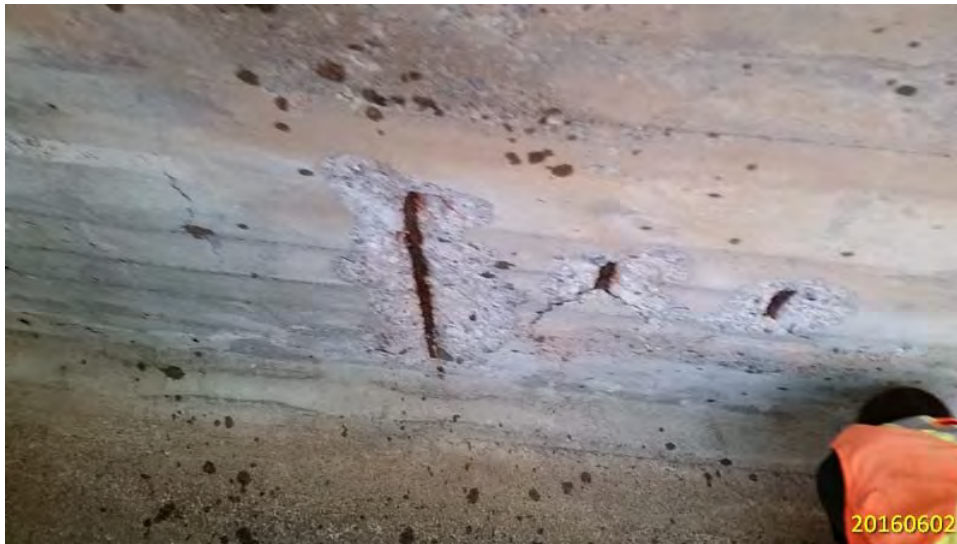
LOCALIZED DELAMINATION WITH EXPOSED CORRODED REBAR IN WEST DECK SOFFIT
