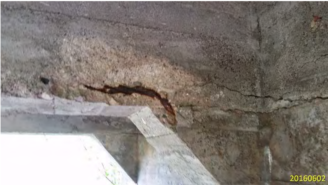
EXPOSED CORRODED REBAR IN SOUTHEAST INTERIOR BEAM
