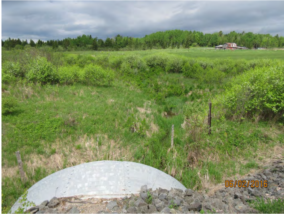
LOOKING WEST UPSTREAM FROM STRUCTURE
