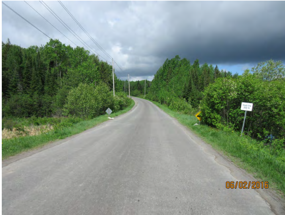
LOOKING WEST ACROSS STRUCTURE
