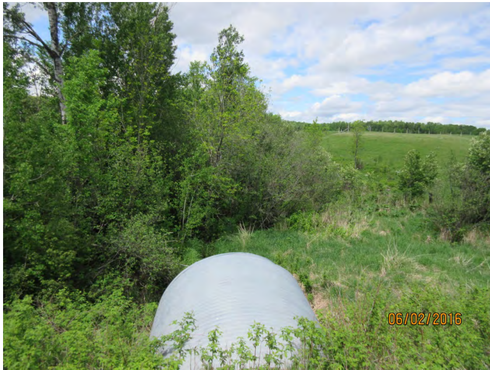
LOOKING UPSTREAM FROM CULVERT
