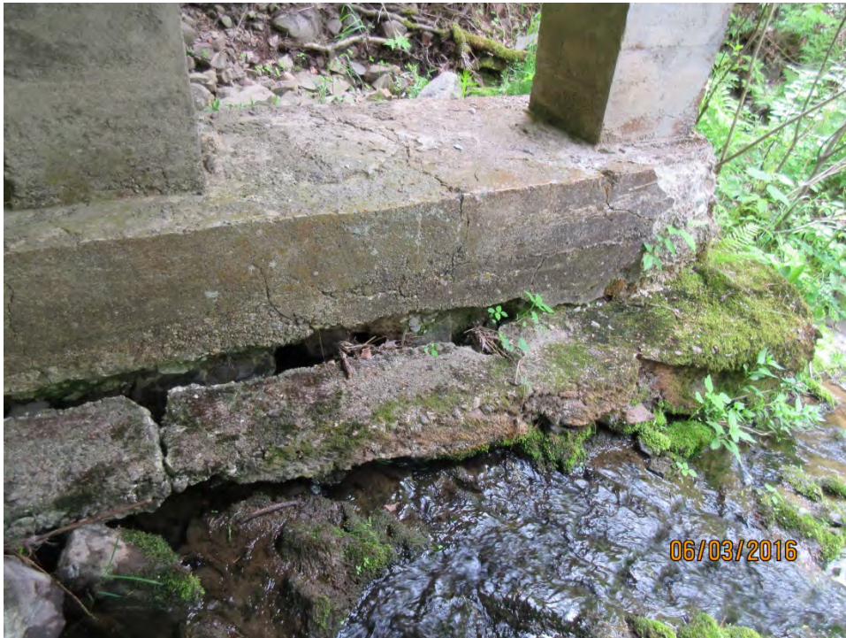
BROKEN CONCRETE FOOTING WITH MODERATE TO SEVERE UNDERMINING
