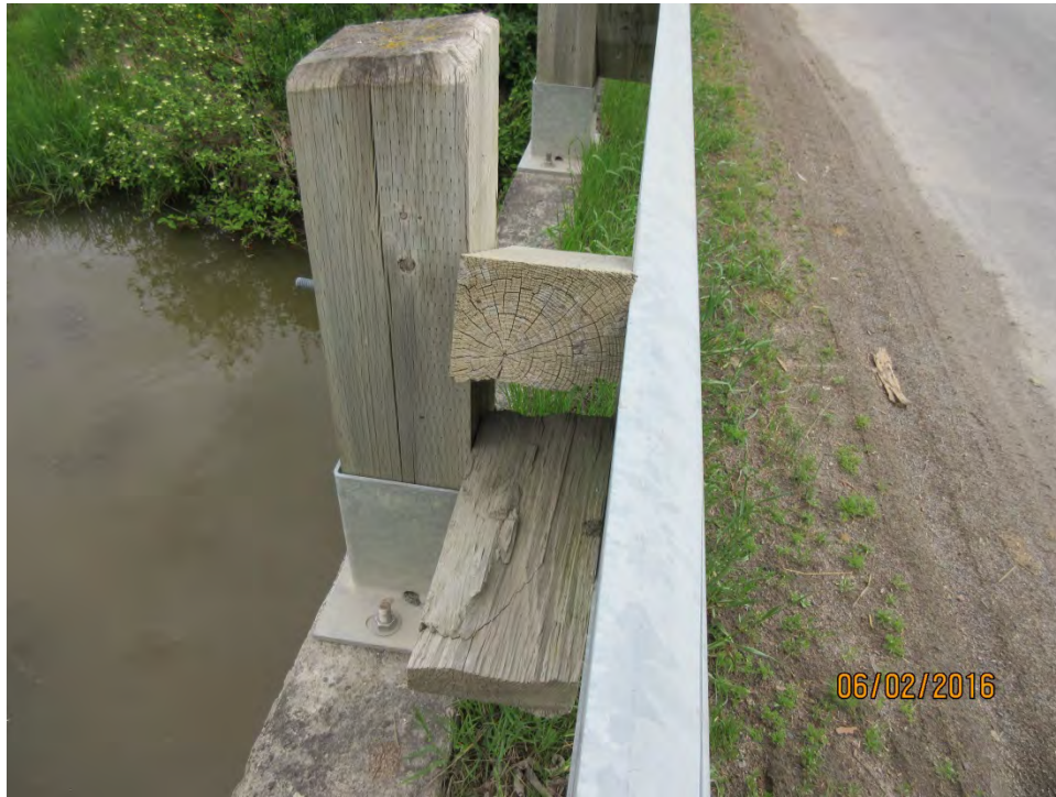
ROTATED AND SPLIT OFFSET BLOCK – NORTH GUARDRAIL
