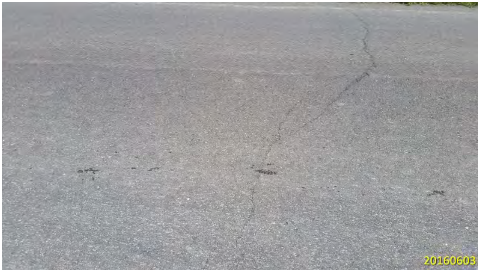
MEDIUM TRANSVERSE CRACK IN SOUTH APPROACH WEARING SURFACE
