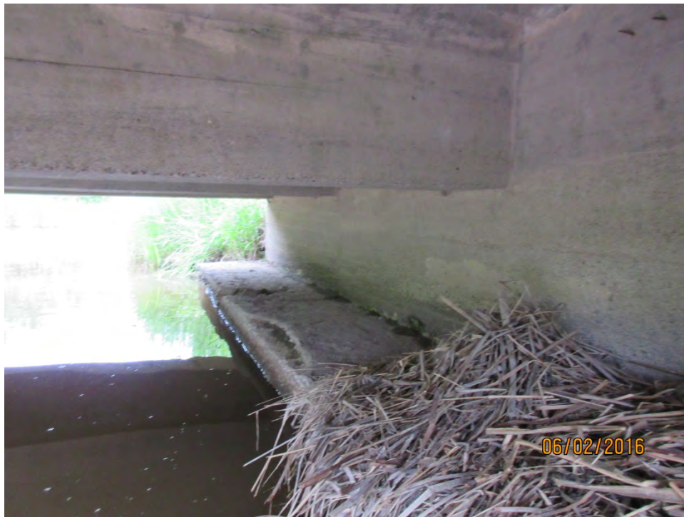
WEST ABUTMENT WALL AND FOOTING – SEVERE DELAMINATION OF TOP OF FOOTING
