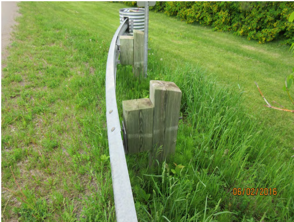
TYPICAL BARREL END TREATMENT
