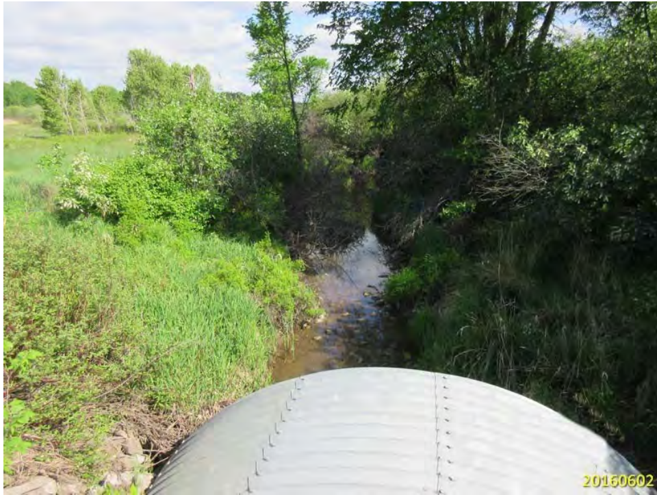
LOOKING NORTH UPSTREAM FROM STRUCTURE
