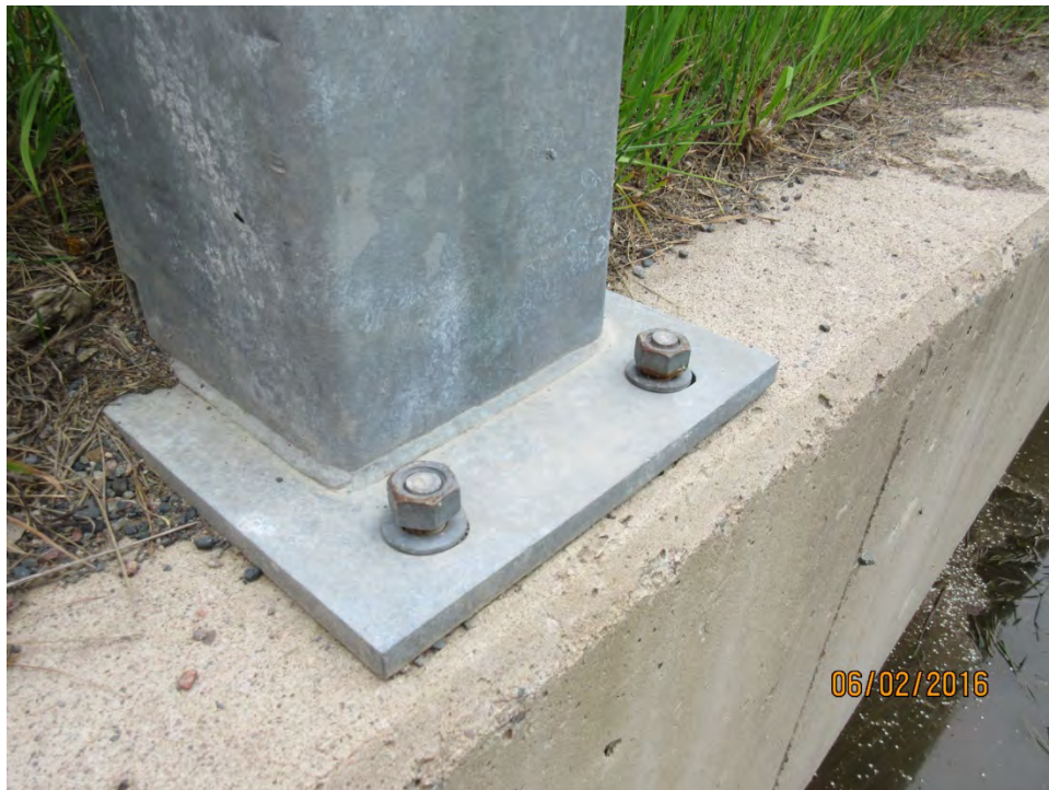
LOOSE NUTS ON BASEPLATE OF EAST GUIDERAIL POST
