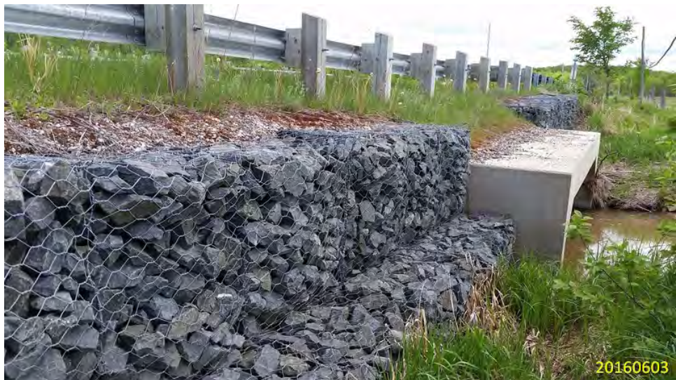
GABION BASKETS ALONG WEST ROADWAY EMBANKMENTS
