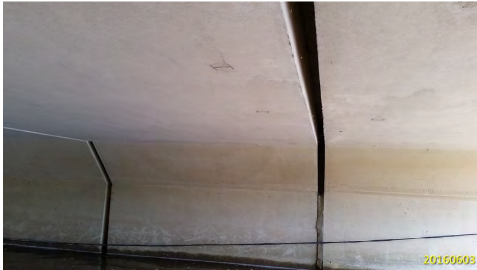
LOSS OF PARGING IN CULVERT BARREL JOINTS
