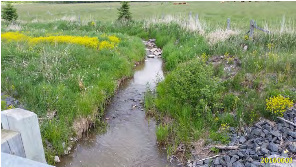
LOOKING UPSTREAM OF STRUCTURE
