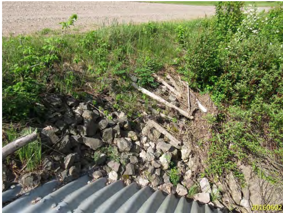
TYPICAL ROCK PROTECTION ON ROADWAY EMBANKMENT
