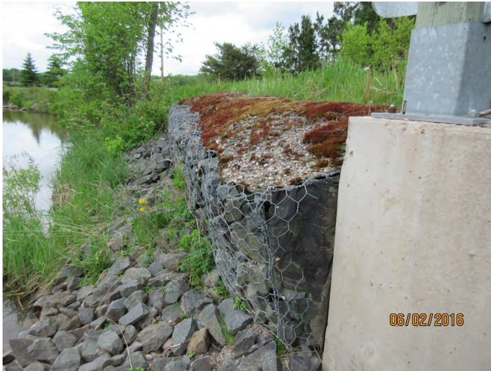
ROTATED GABION BASKET WINGWALL – NORTHWEST WINGWALL
