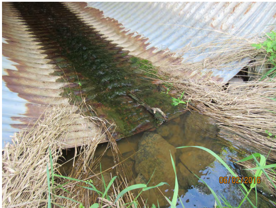
CULVERT INLET WITH MODERATE UNDERMINING
