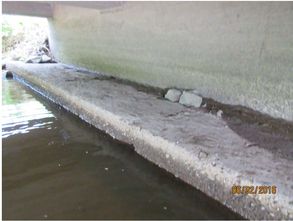
EAST ABUTMENT WALL AND FOOTING – EROSION OF CONCRETE FOOTING
