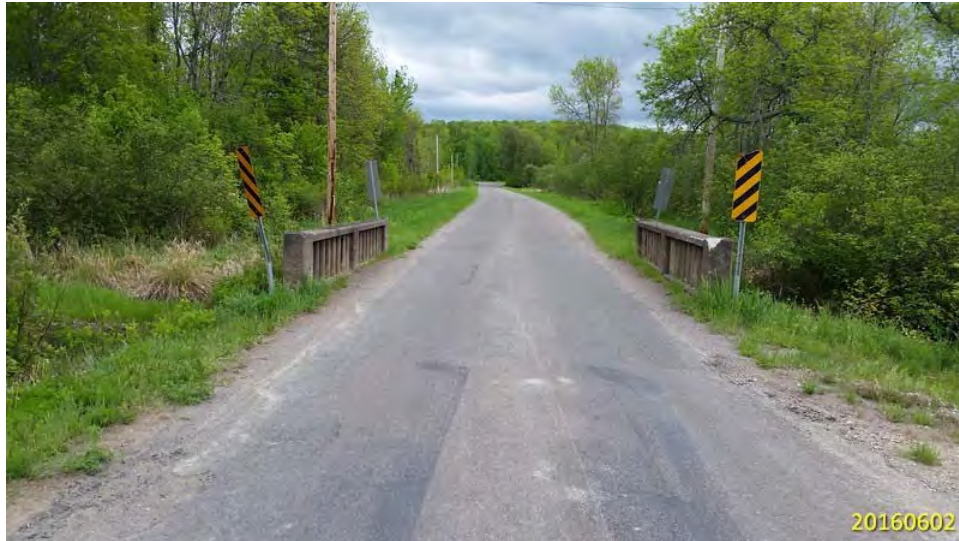
LOOKING SOUTH ACROSS STRUCTURE
