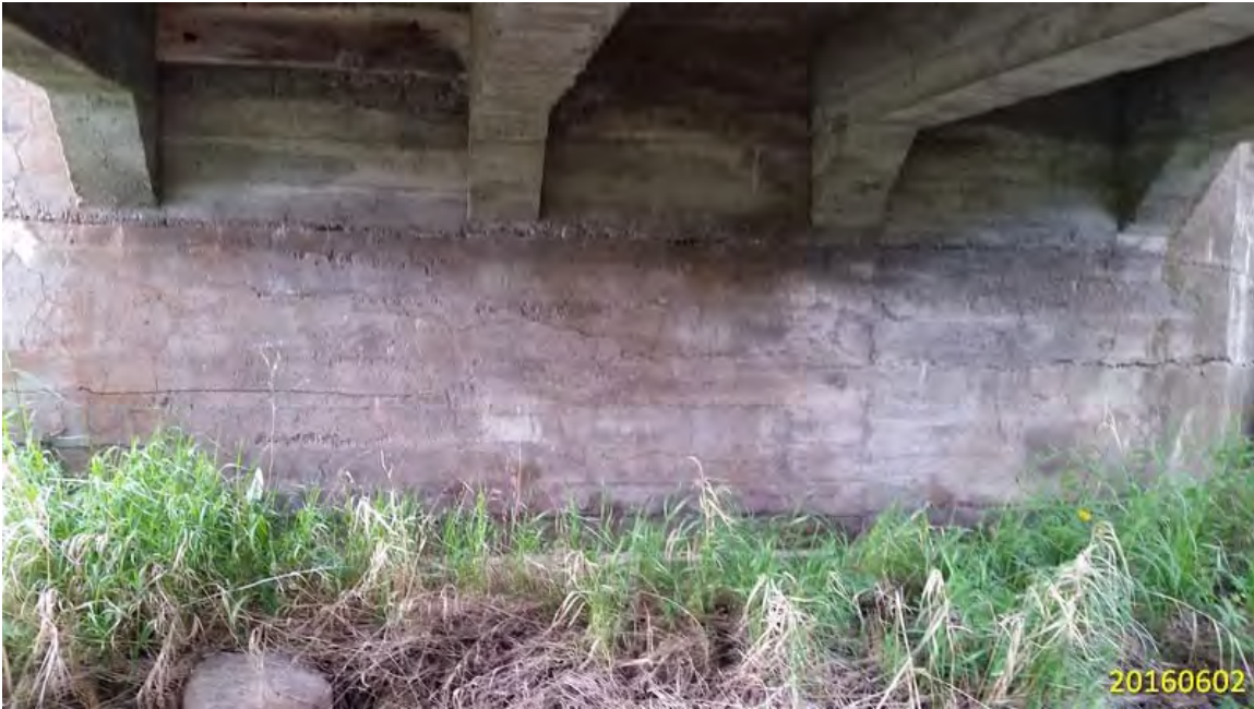
NORTH ABUTMENT WALL – NARROW TO MEDIUM MAP CRACKING, NARROW TO WIDE HORIZONTAL CRACKING AND DELAMINATIONS
