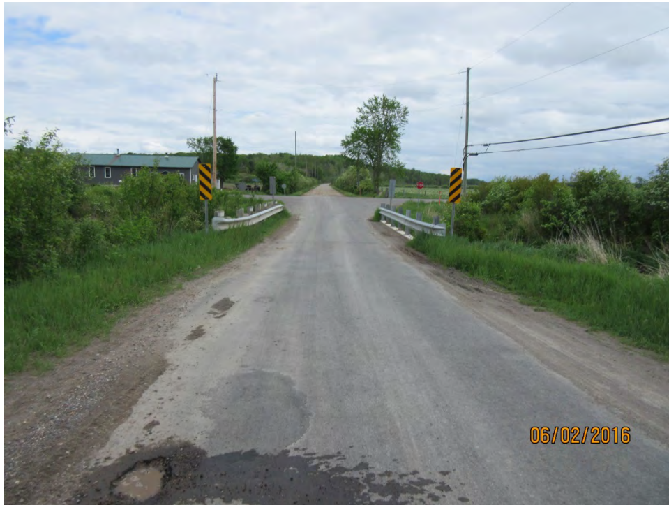
LOOKING EAST ACROSS STRUCTURE
