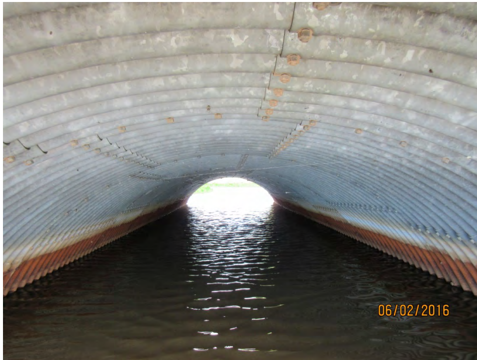
LOOKING WEST THROUGH CULVERT BARREL
