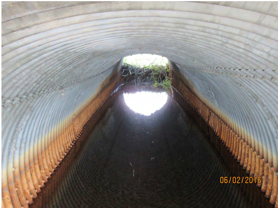
LOOKING NORTH THROUGH CULVERT BARREL – SIGNIFICANT SAG IN BARREL ALONG ITS LENGTH
