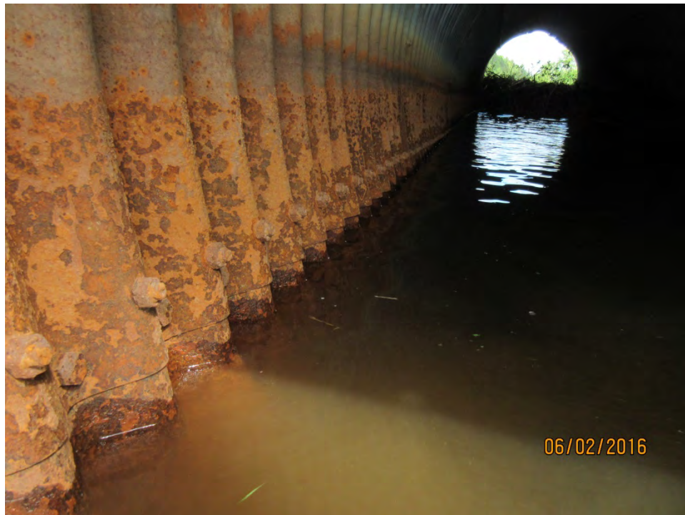
LIGHT TO MODERATE CORROSION OF CULVERT BARREL WITH FLAKING AT WATERLINE
