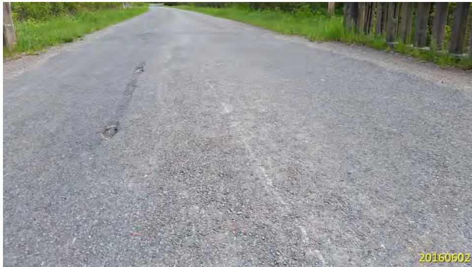
DECK WEARING SURFACE WITH LIGHT WEAR, ABRASIONS AND LOCALIZED POTHOLES
