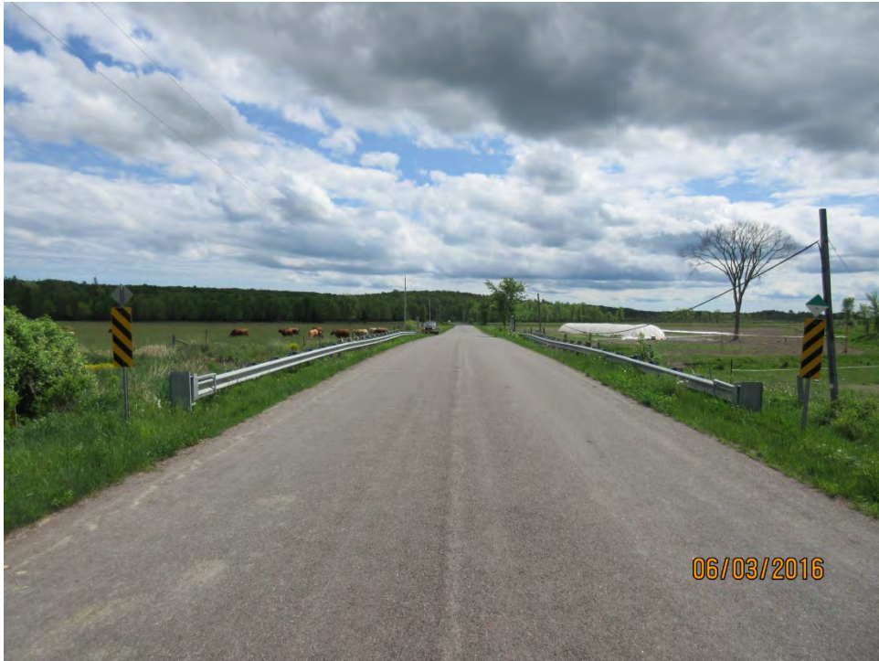
LOOKING SOUTH ACROSS STRUCTURE
