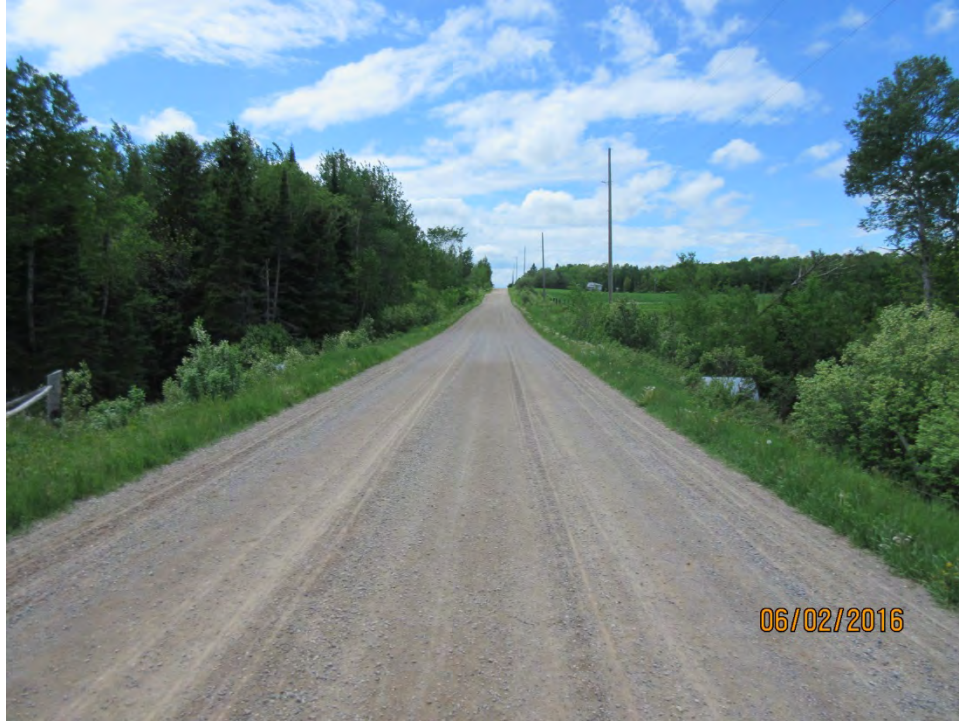
LOOKING WEST ACROSS STRUCTURE
