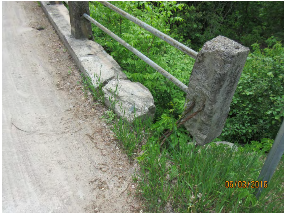
BROKEN SECTION OF CURB AND MISSING SECTION OF RAILING POST IN THE NORTHWEST CORNER
