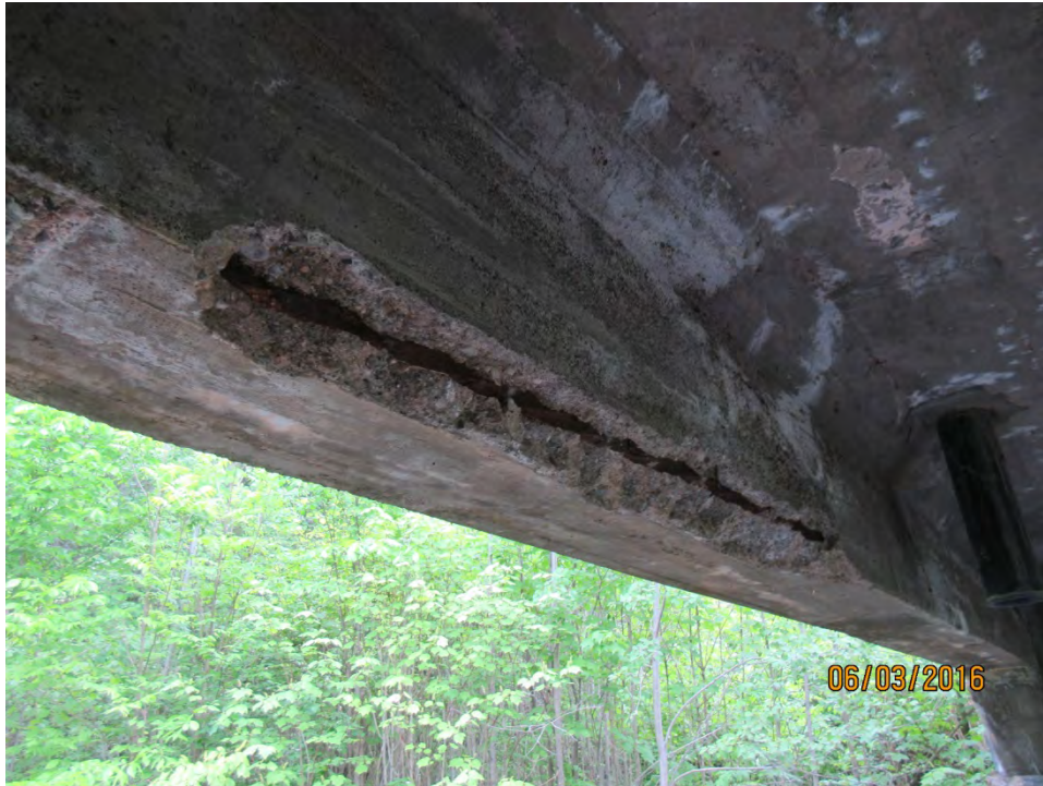
EXPOSED CORRODED REBAR IN EAST EXTERIOR BEAM'S NORTH SPAN
