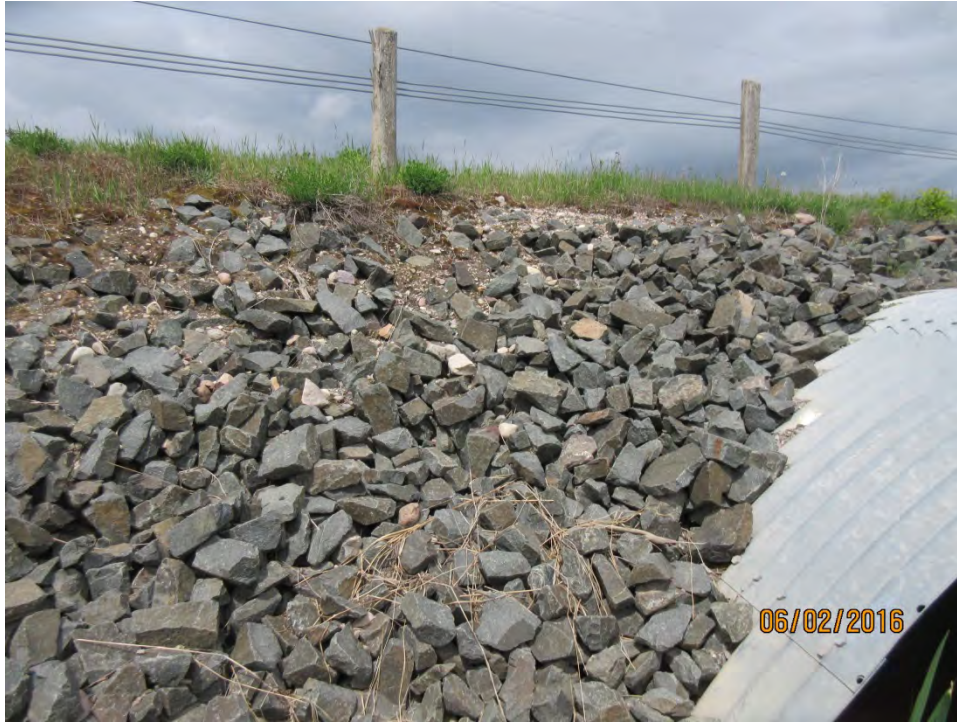
TYPICAL ROCK PROTECTION AND EMBANKMENT
