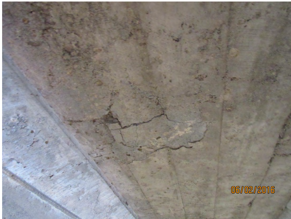
LOCALIZED MEDIUM TO WIDE CRACKING OF INTERIOR DECK SOFFIT AT THE EAST ABUTMENT
