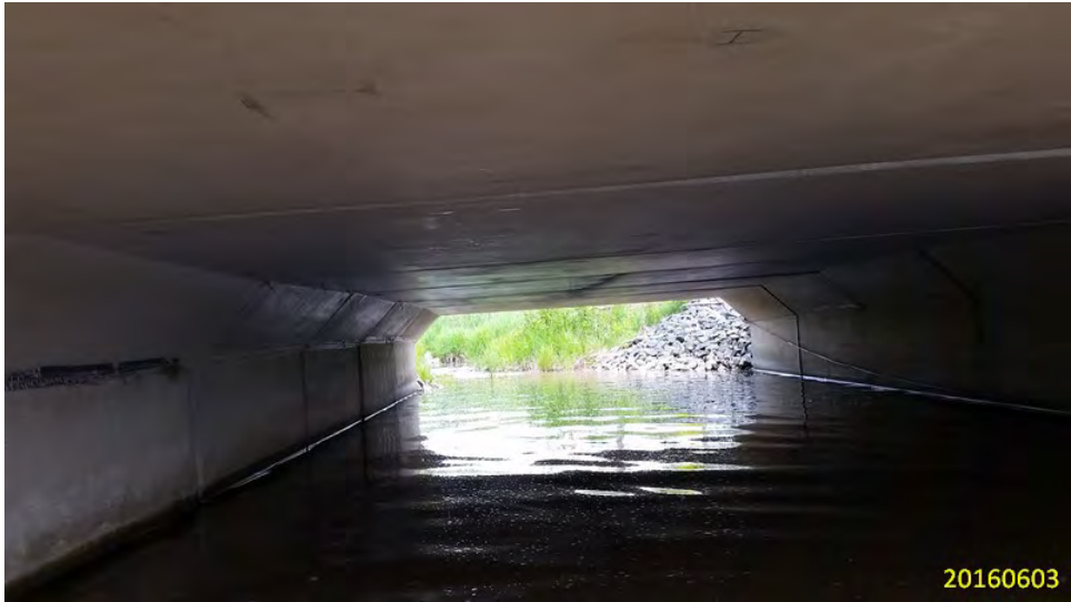
LOOKING EAST THROUGH BARREL
