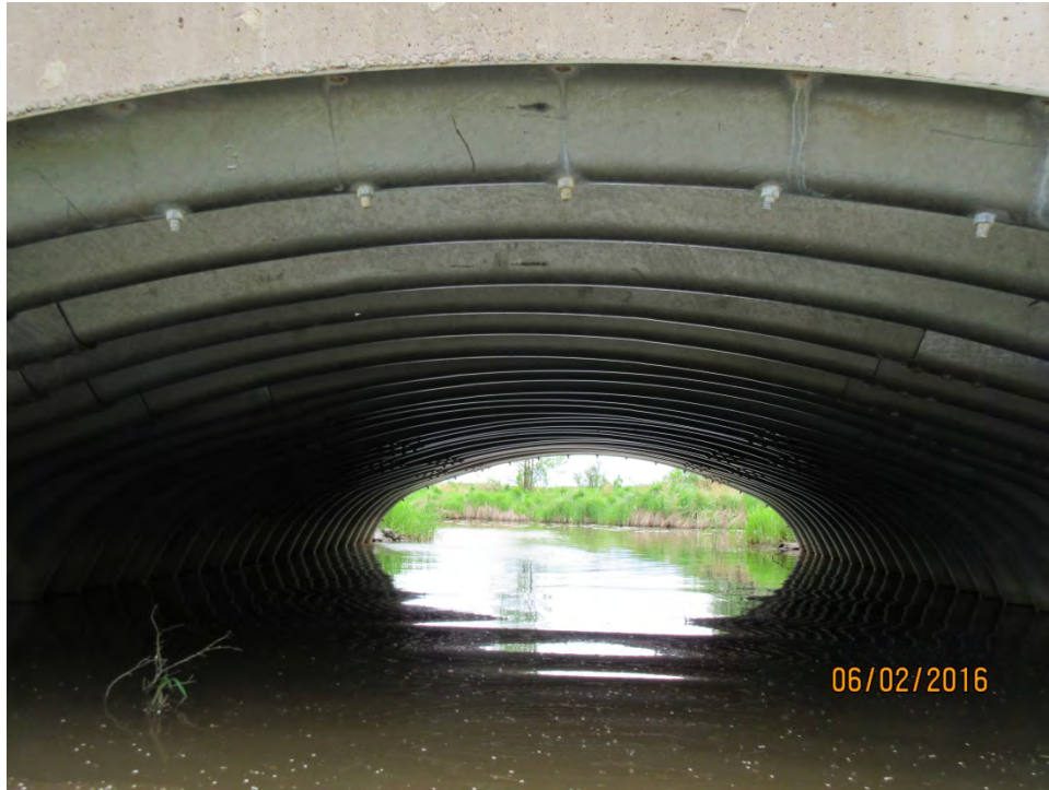
LOOKING WEST THROUGH CULVERT BARREL
