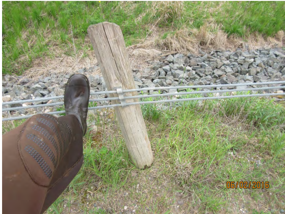
BROKEN GUIDERAIL POST ALONG EAST GUIDERAIL
