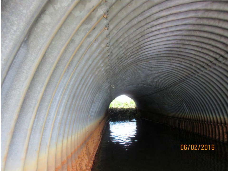
LOOKING NORTH THROUGH CULVERT BARREL
