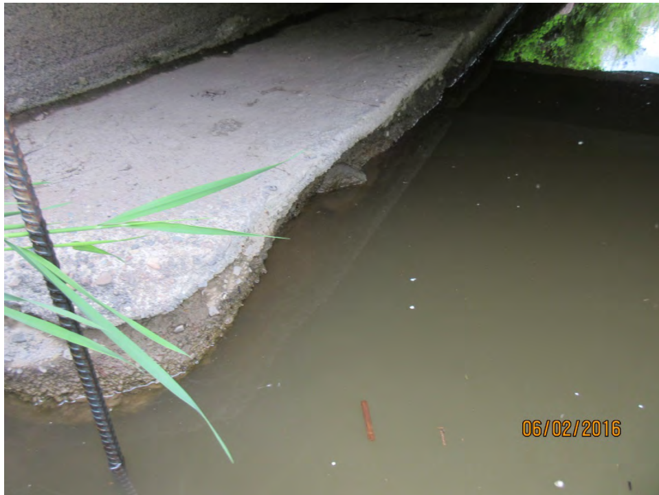
CONCRETE EROSION AND LARGE SPALL IN FOOTING
