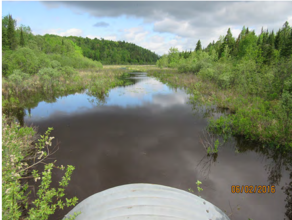
LOOKING NORTH UPSTREAM FOR STRUCTURE
