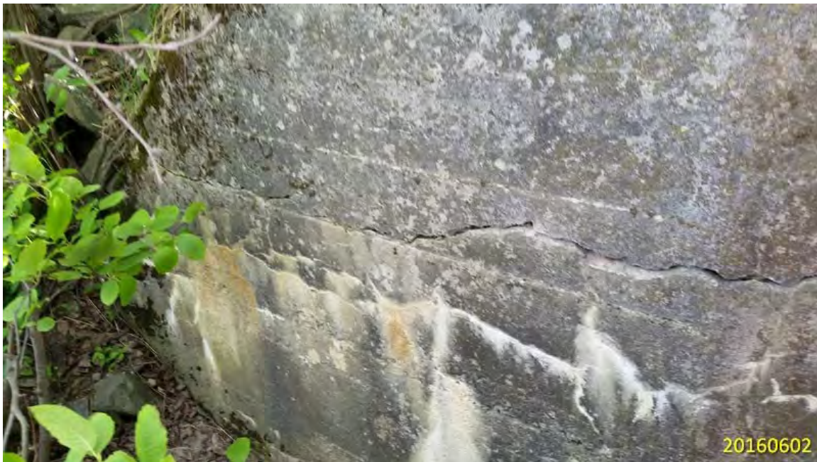
SOUTHEAST WINGWALL – NARROW TO MEDIUM MAP CRACKING AND WIDE HORIZONTAL CRACK
