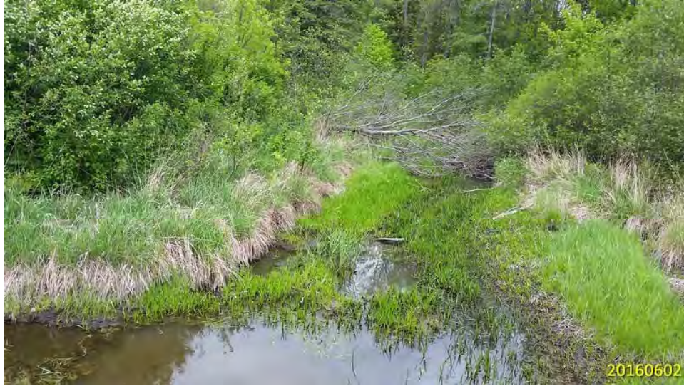
UPSTREAM FROM BRIDGE, TREE OBSTRUCTING WATERWAY
