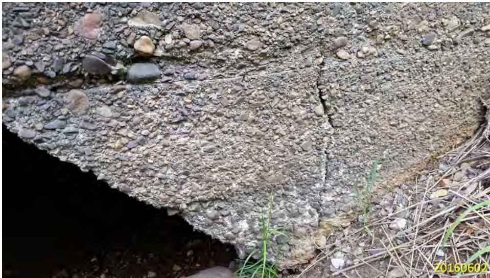
MEDIUM TO WIDE CRACK IN SOUTHWEST BEAM HAUNCH
