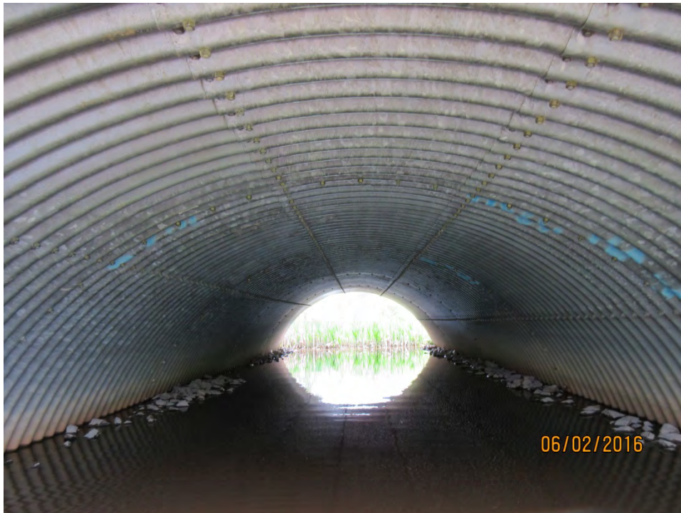
LOOKING EAST THROUGH CULVERT BARREL
