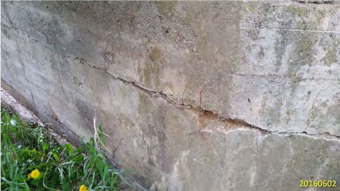
NORTH ABUTMENT AND NORTHEAST WINGWALL - LOCALIZED SPALL WITH DELAMINATIONS
