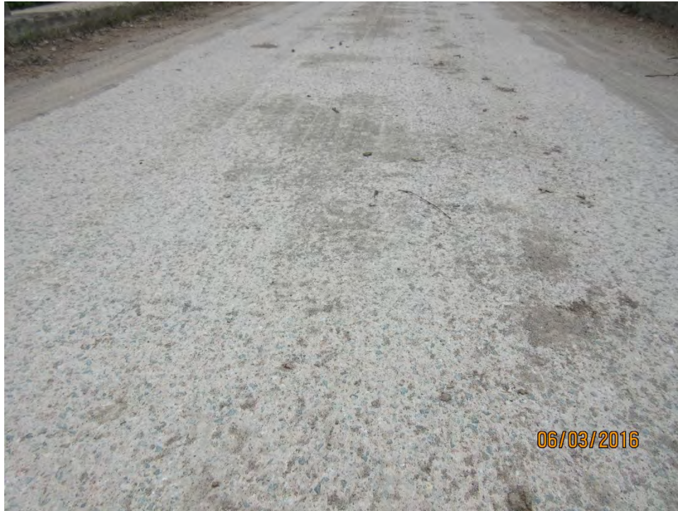
BRIDGE DECK WEARING SURFACE – LIGHT TO MODERATE SCALING AND ABRASIONS
