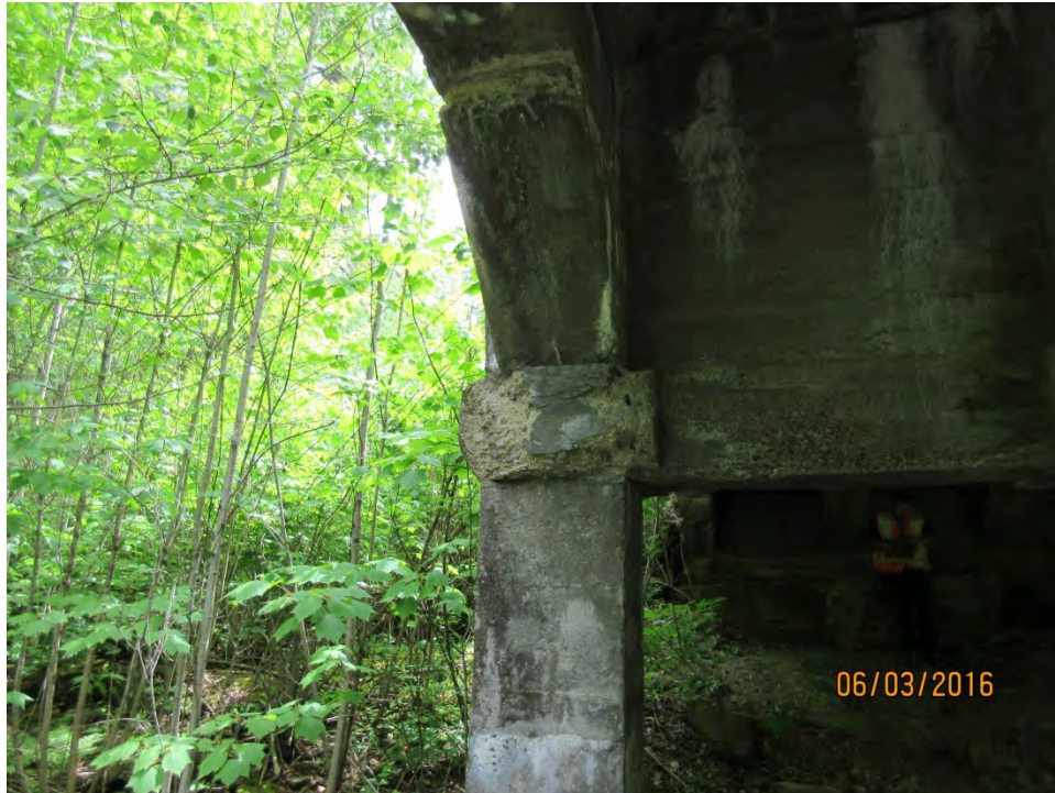
CONCRETE SPALL AND DISINTEGRATION OF SOUTH PIER
