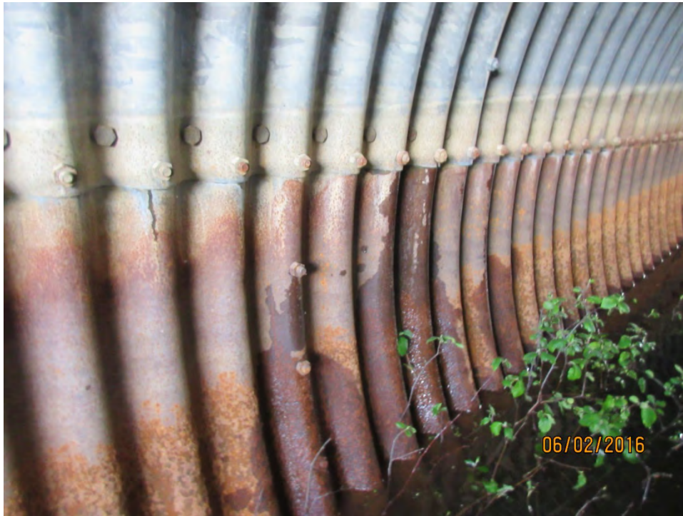
WATER INFILTRATION AT BOLT JOINT IN NORTH SECTION OF WEST WALL
