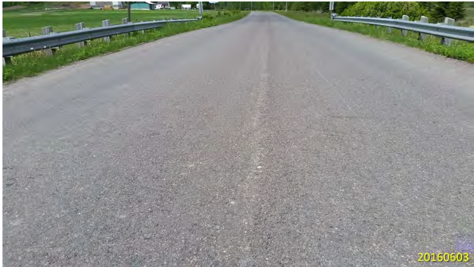
DECK WEARING SURFACE – FACING NORTH
