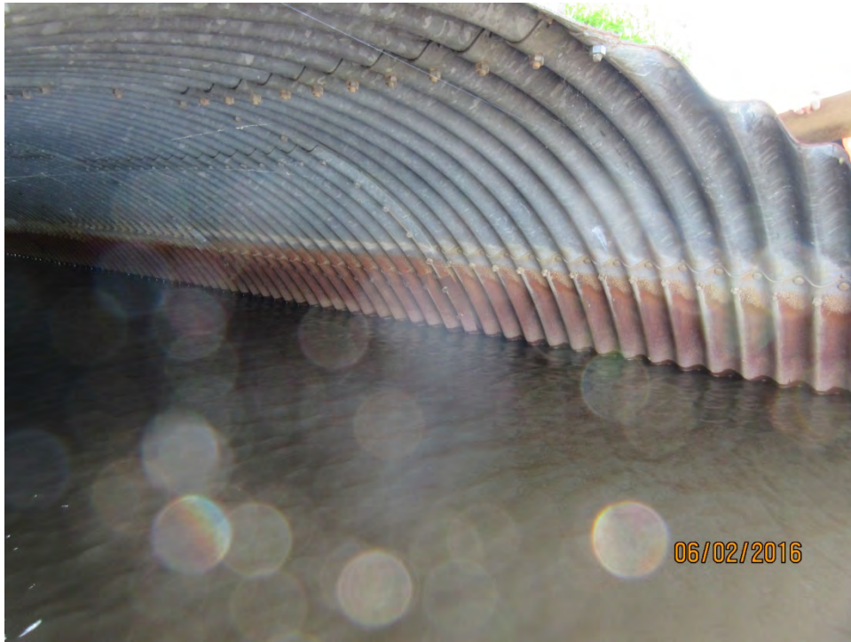
LIGHT TO MODERATE CORROSION OF CULVERT BARREL AT WATERLINE
