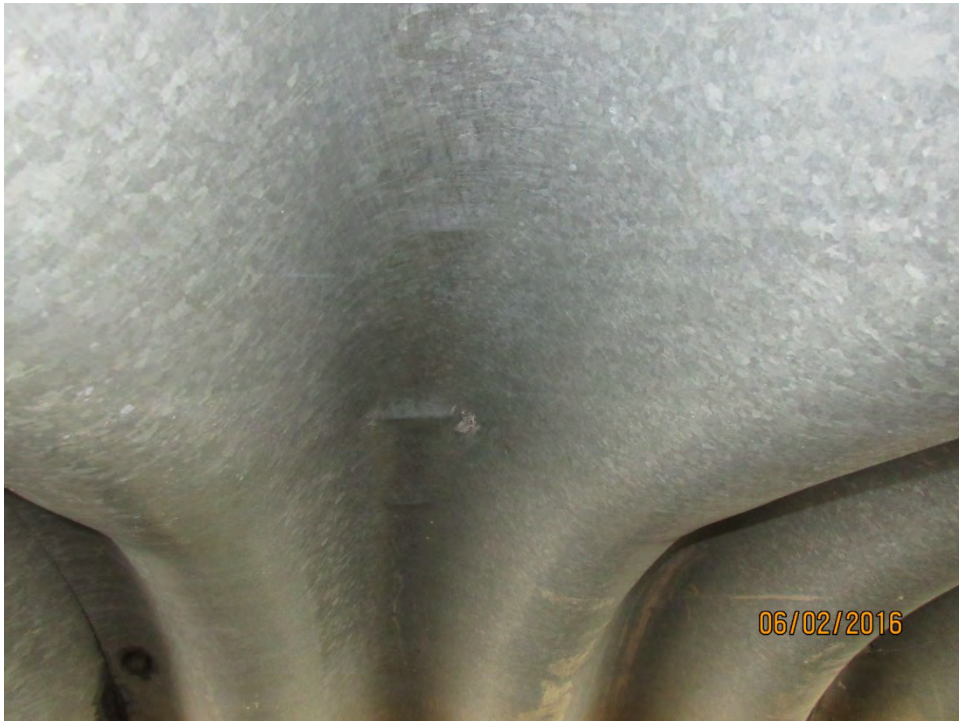
LOCALIZED INDENTATIONS IN THE RIBS OF THE CULVERT BARREL
