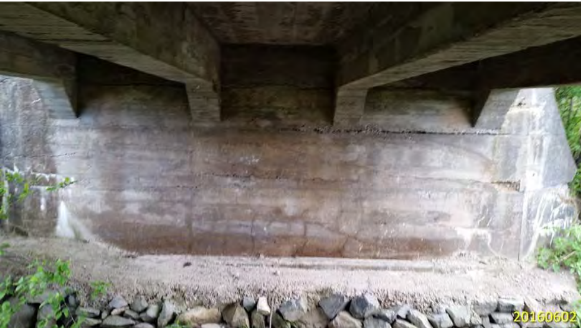
SOUTH ABUTMENT WALL – NARROW TO MEDIUM MAP CRACKING, NARROW TO WIDE HORIZONTAL CRACKING AND DELAMINATIONS
