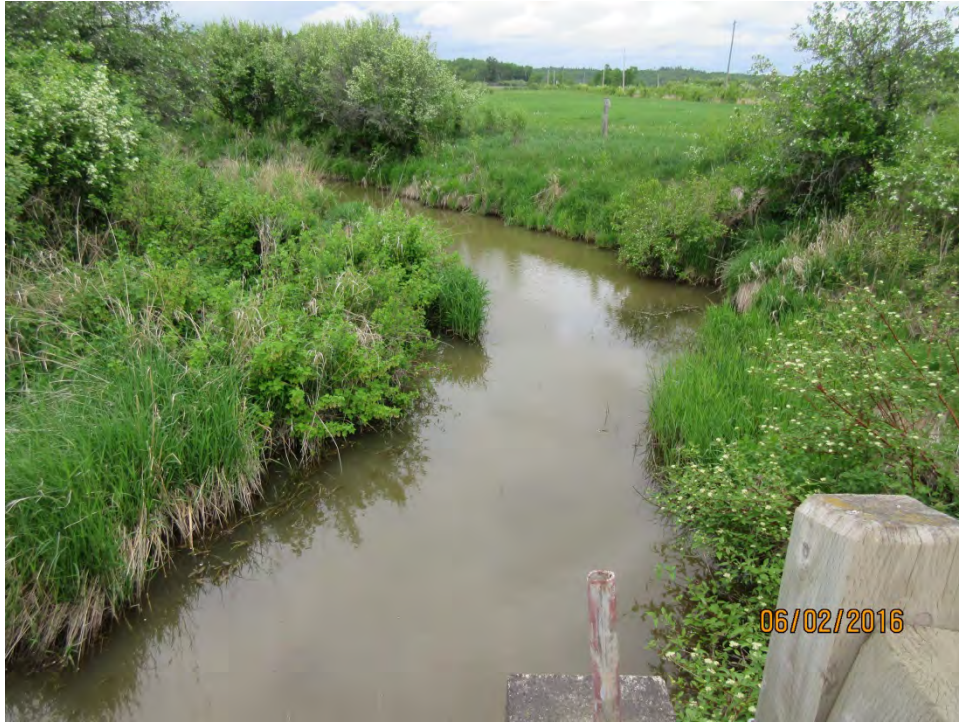
LOOKING NORTH, UPSTREAM OF STRUCTURE
