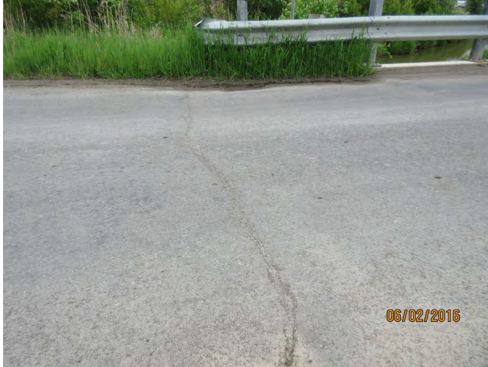
MODERATE TO WIDE TRANSVERSE CRACK IN EAST APPROACH
