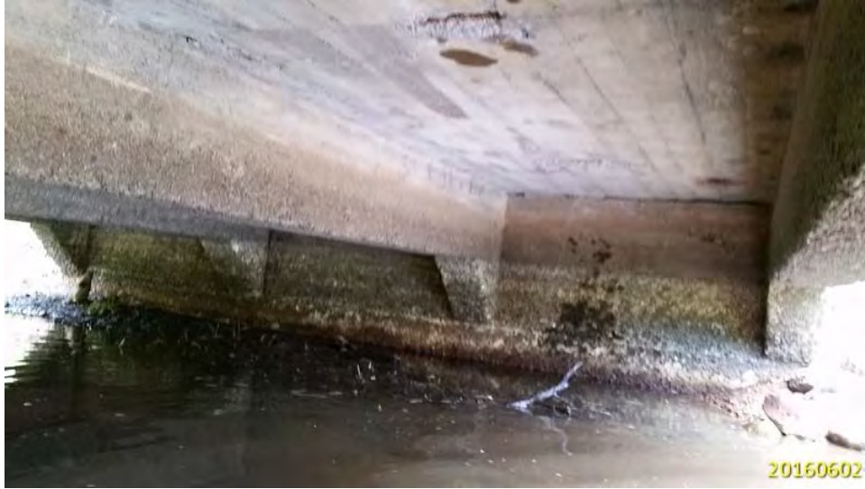
SOUTH ABUTMENT WITH MODERATE TO SEVERE EROSION
