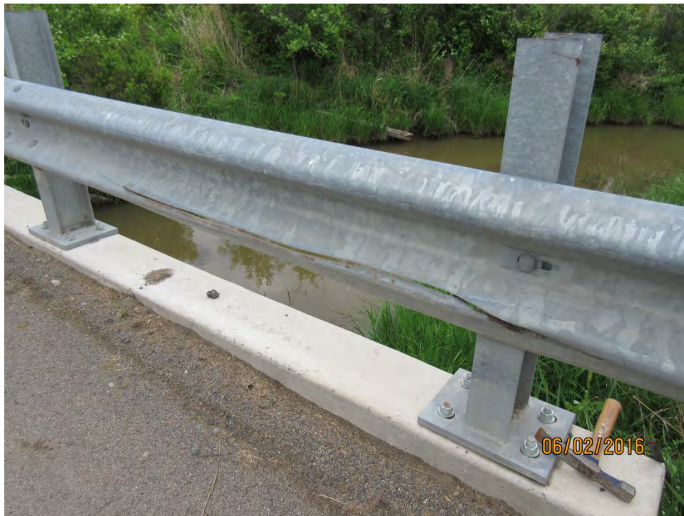
LARGE CUT IN THE SOUTHWEST GUIDERAIL
