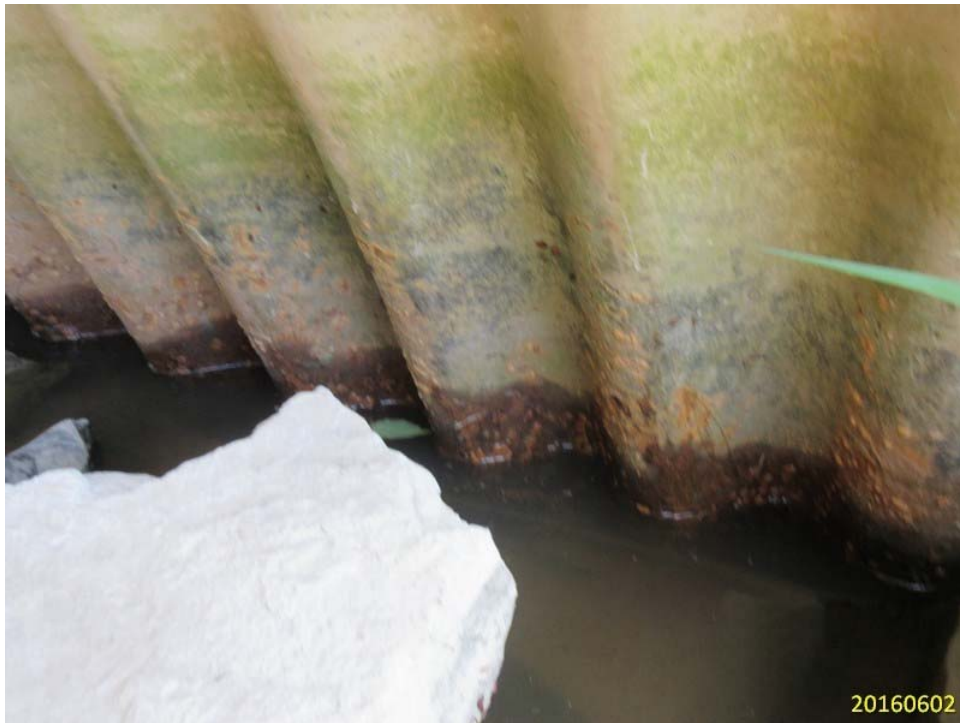
LIGHT STAINING AND BLISTERING OF COATING AT WATERLINE – SOUTHEAST QUADRANT
