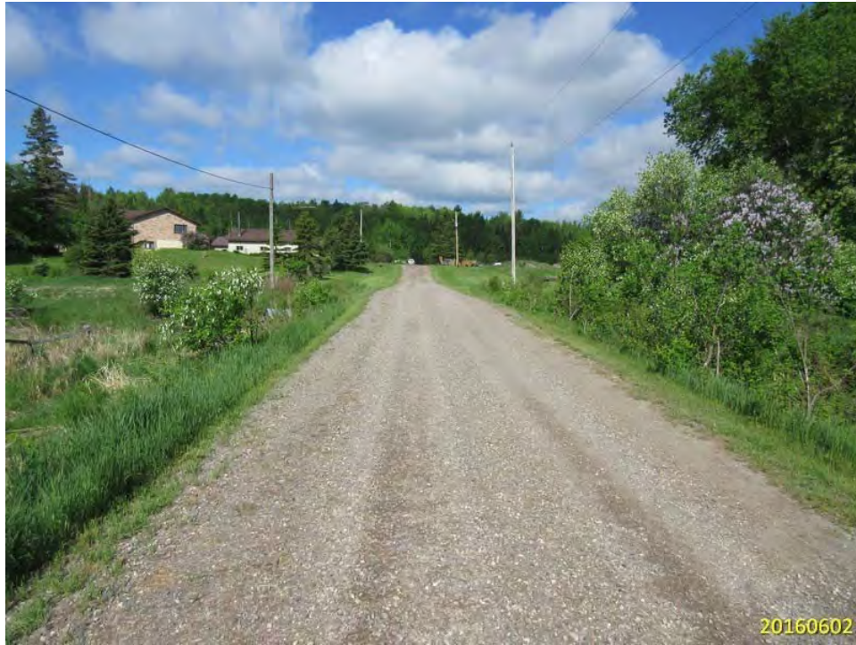
LOOKING WEST ACROSS STRUCTURE
