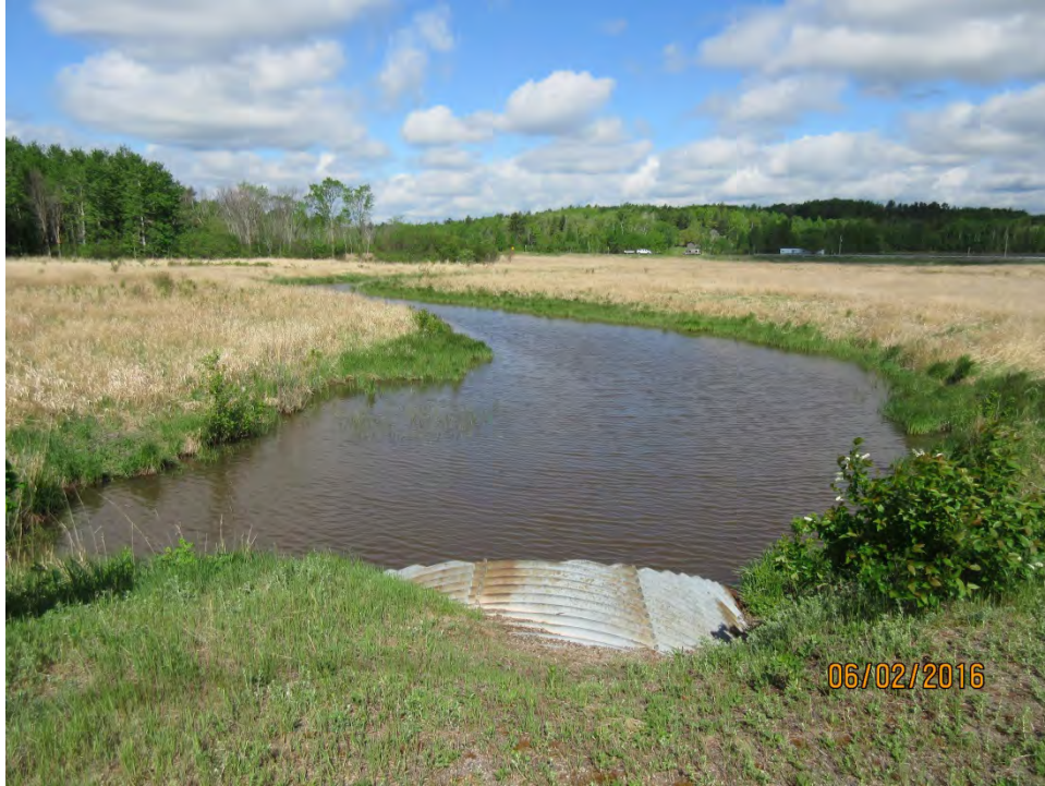
LOOKING WEST UPSTREAM FROM STRUCTURE
