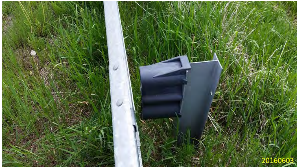
GUIDERAIL POST MISSING BOLT
