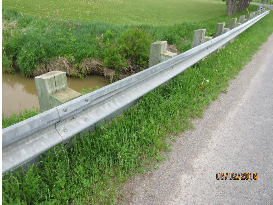
SCRAPE DAMAGE TO EAST GUIDERAIL
