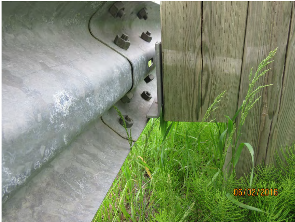
MEDIUM TO WIDE SPLITS AND CHECKS IN APPROACH POSTS AND OFFSET BLOCKS
