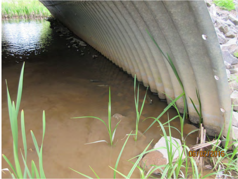
LIGHT STAINING OF CULVERT BARREL AT WATERLINE AND LOSS OF ARMORING STONE AT INLET
