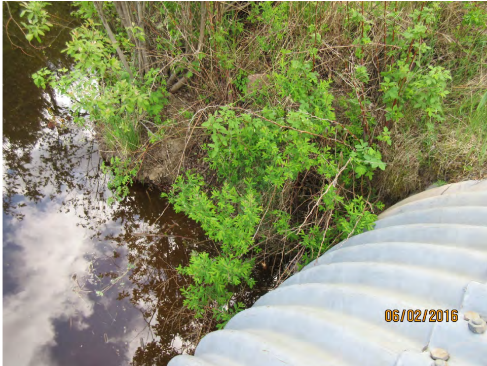
SEVERE EROSION AND SCOUR AT CULVERT INLET/NORTHEAST QUADRANT
