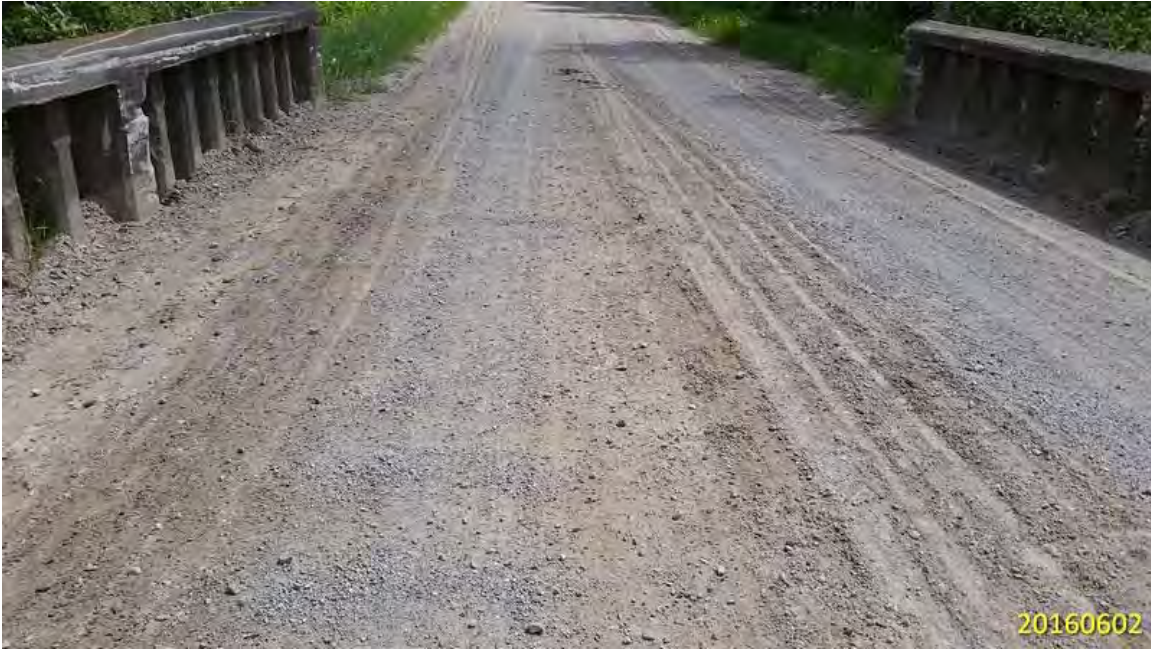
GRAVEL WEARING SURFACE – BUILDUP OF GRAVEL ON BRIDGE DECK AND LIGHT WASHBOARD
