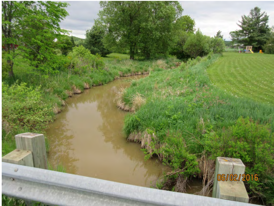
LOOKING EAST UPSTREAM FROM STRUCTURE
