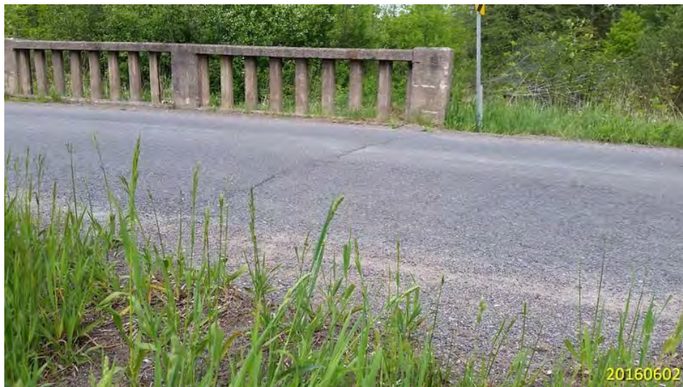
SETTLEMENT OF SOUTH APPROACH AND CRACKING OF WEAR SURFACE AT END OF BRIDGE DECK
