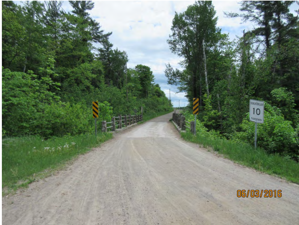
LOOKING SOUTH ACROSS STRUCTURE
