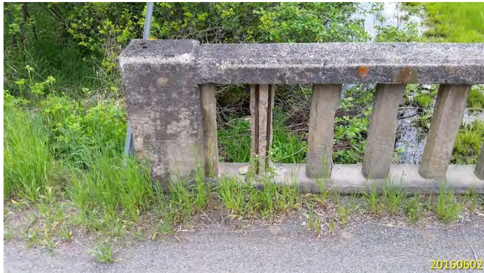
TYPICAL RAILING SYSTEM WITH EXPOSED REBAR (SOUTHWEST QUADRANT)
