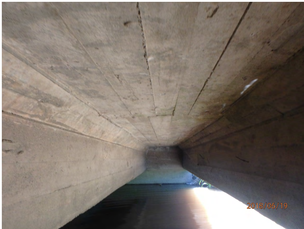
Typical T-beam arrangement
