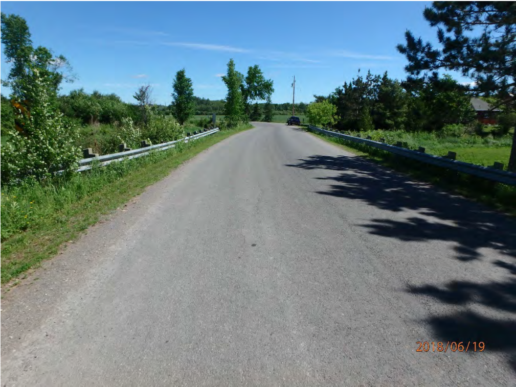
Hazard marker obstructed by vegetation
