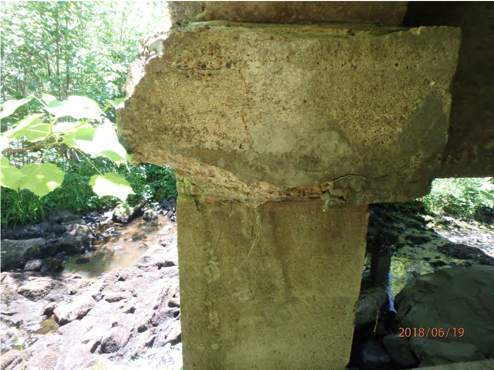
Exposed Rebar on east beam at abutment
