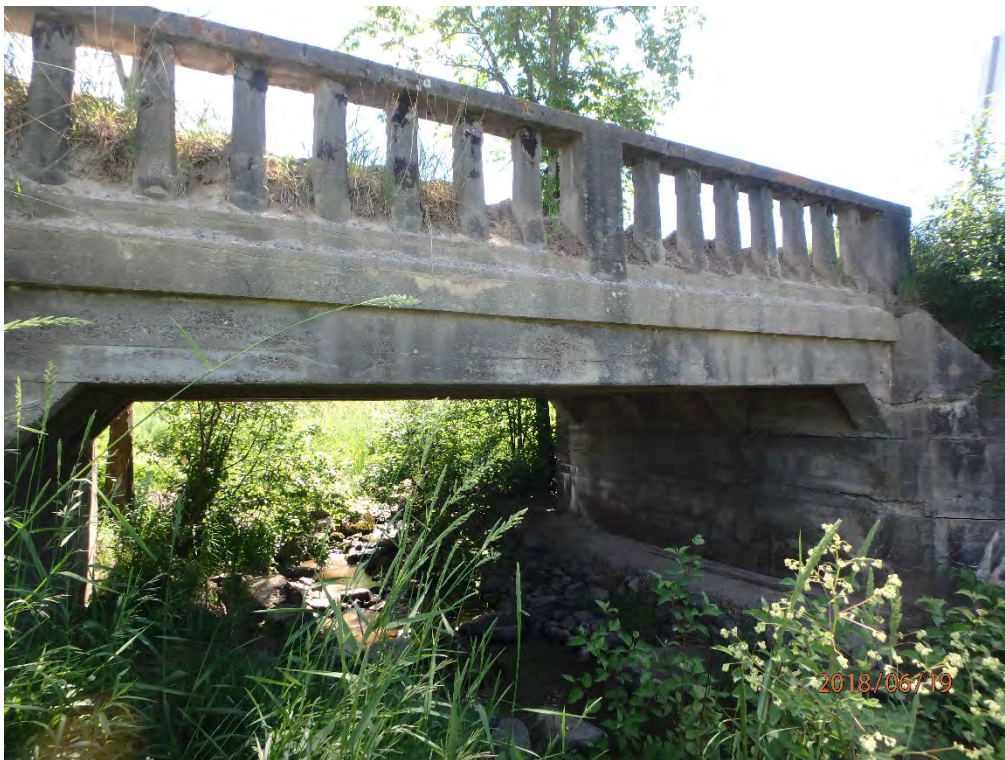
South abutment wall with narrow to wide horizontal cracks, map cracking and delamination.
