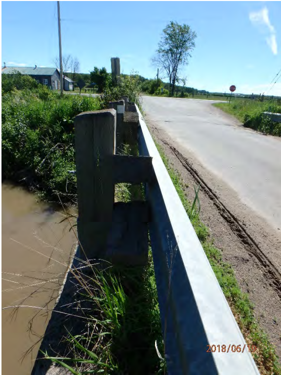
Broken and rotated offset block
