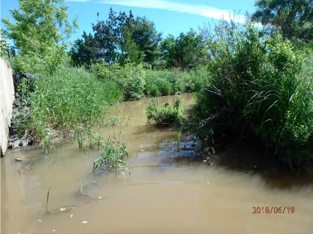
Downstream of Bridge
