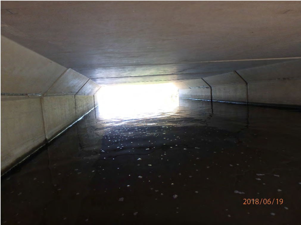
Looking west through barrel
