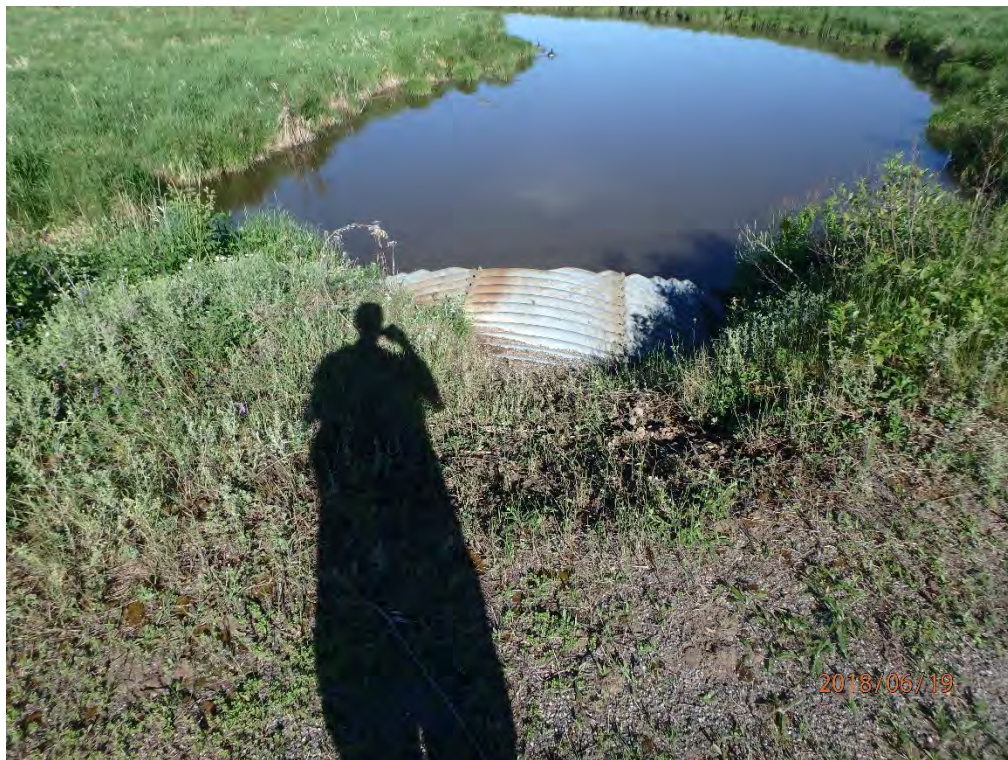
Looking west upstream of culvert
