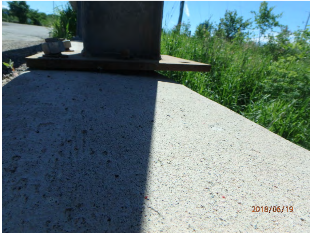
Gap under guiderrail baseplate
