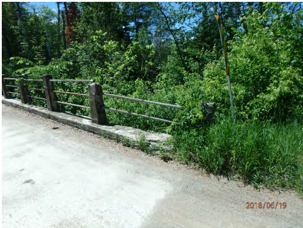
Broken missing railing post. Damaged pipe rails
