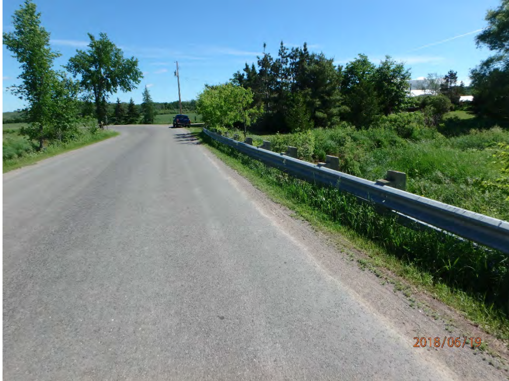
Scraped Guiderail along east side
