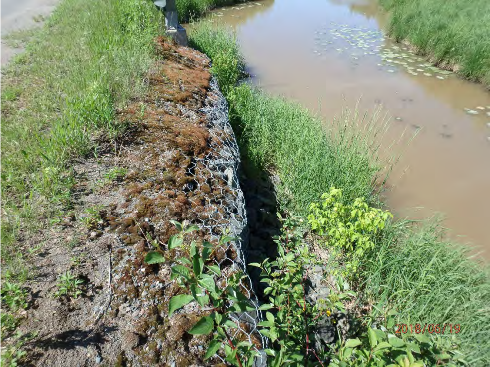
Gabion along the northwest approach
