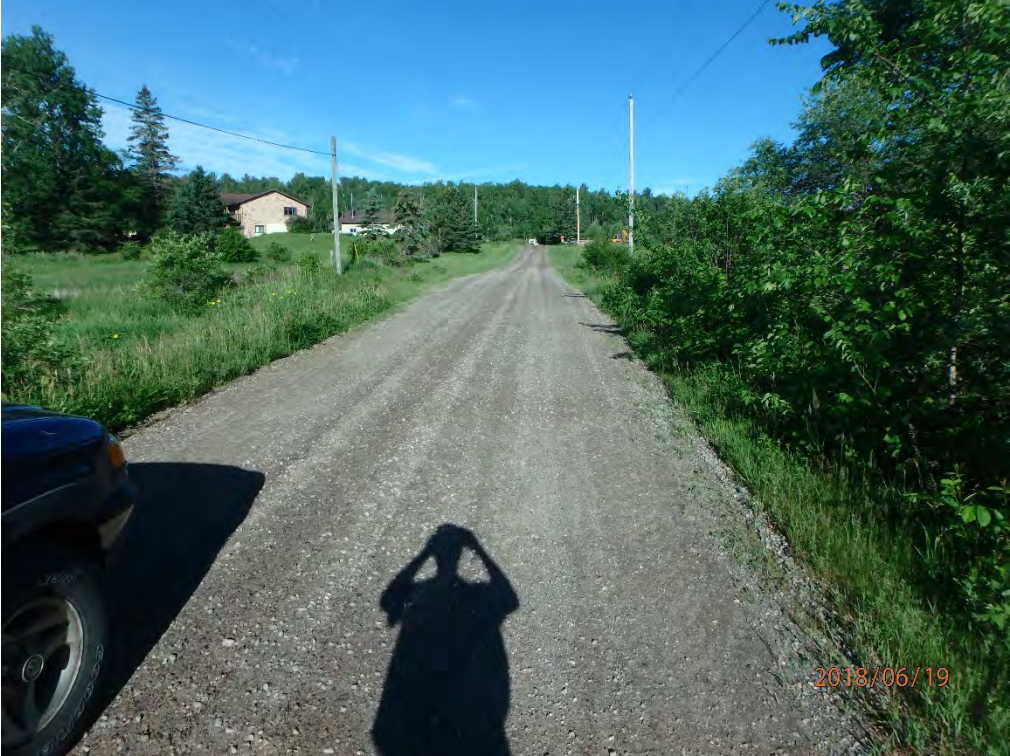
East across the culvert
