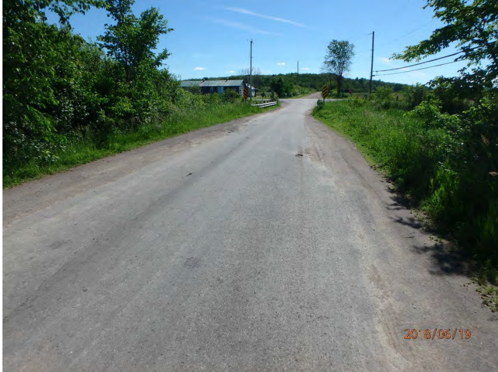
East across the bridge
