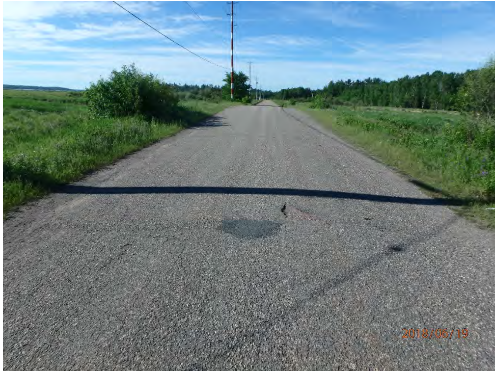
South across the culvert
