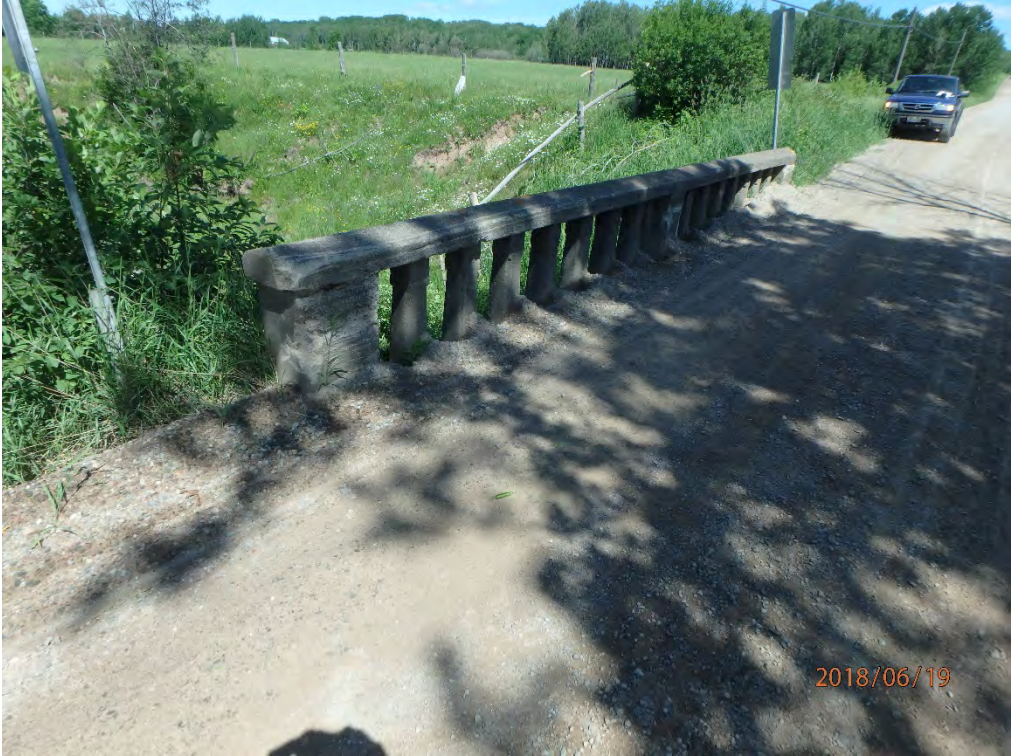
Damage to guard due to impact and buildup of gravel below guard
