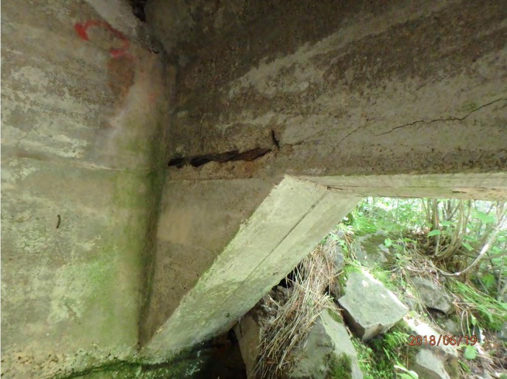
Exposed Rebar on east beam at abutment
