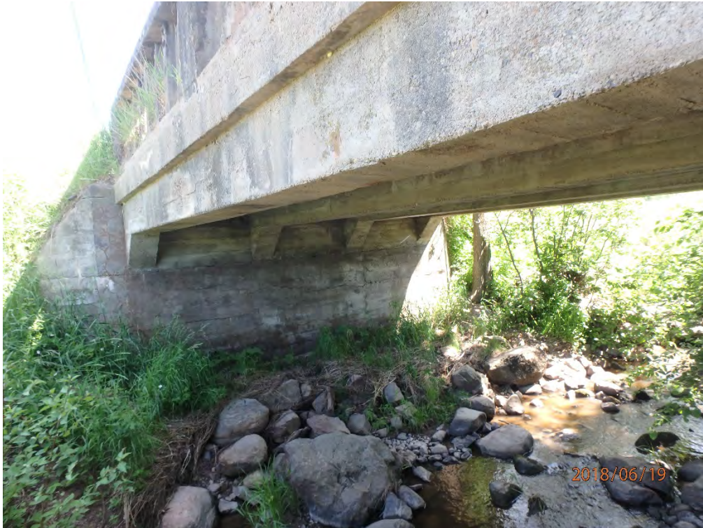
North abutment wall with narrow to wide horizontal cracks, map cracking and delamination.
