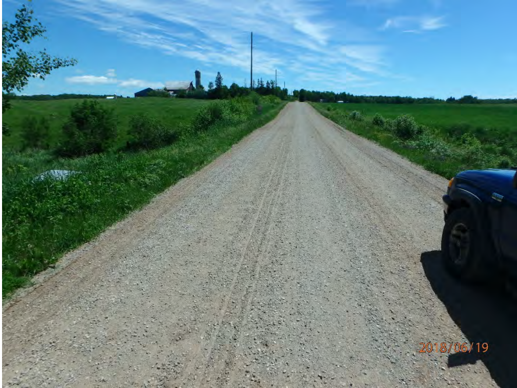
East Across culvert
