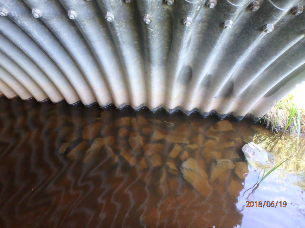
Light staining at waterline
