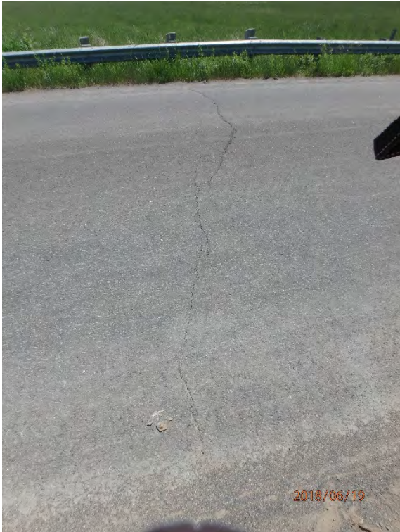
Transverse crack in the wearing surface
