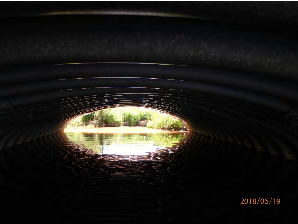
East through the Culvert
