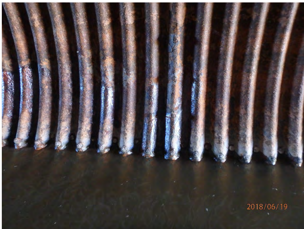
Culvert is rusting and flaking off. Water infiltrating through perforations in metal culvert.
