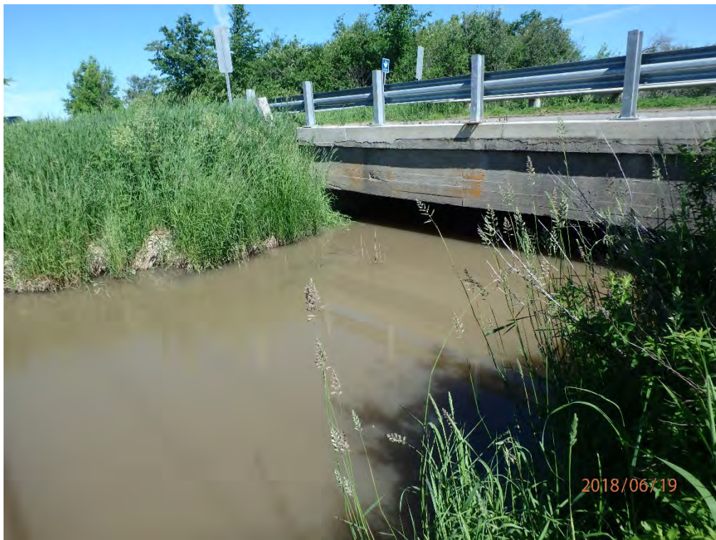
South Elevation of bridge
