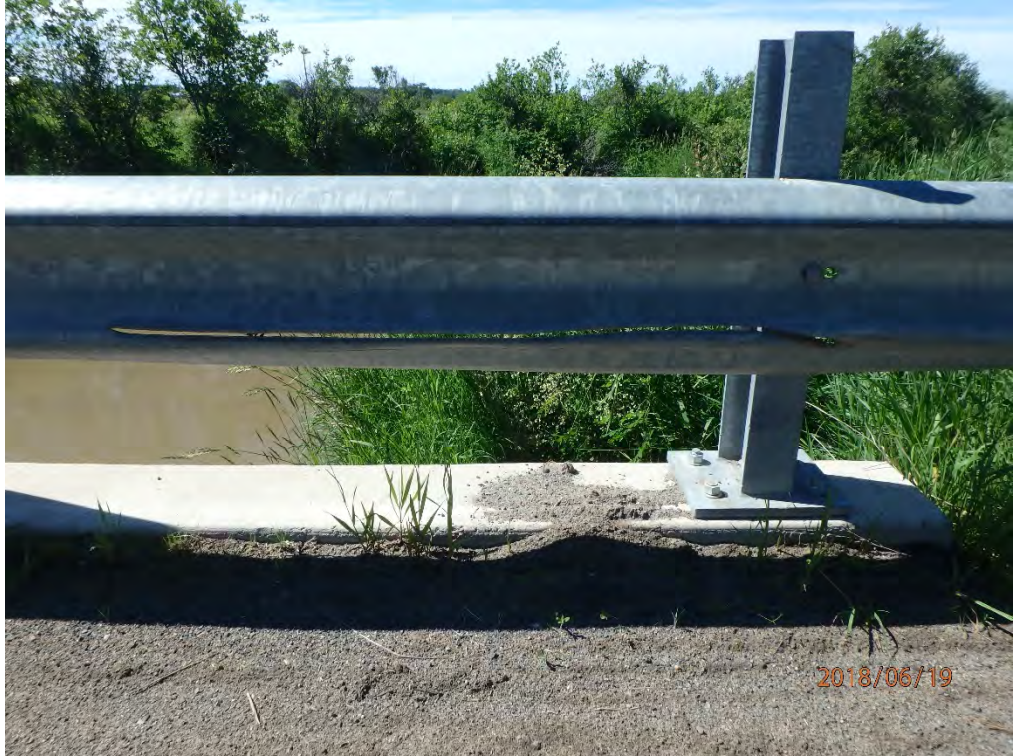
Damaged Guiderail along south side
