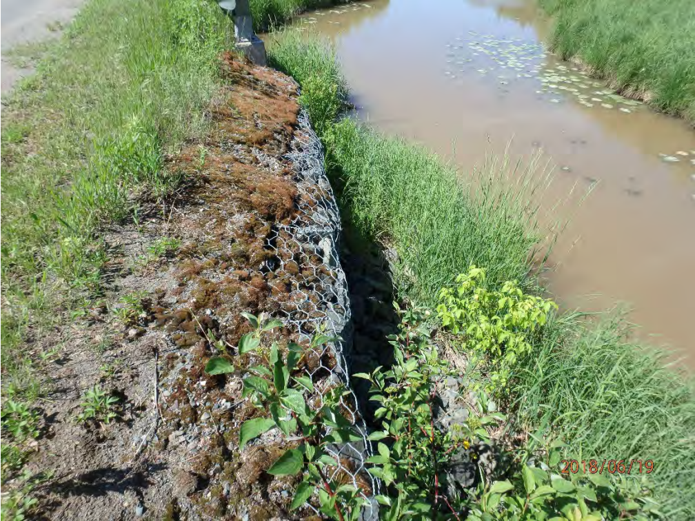
Gabion along the northwest approach
