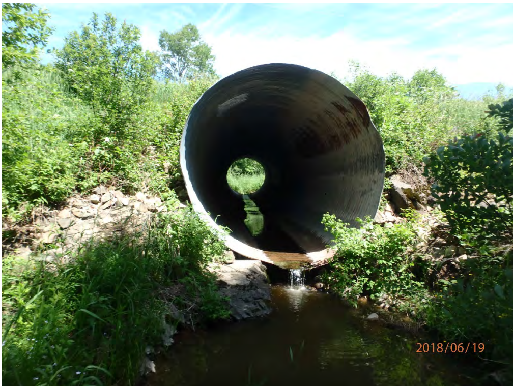
South end of culvert looking at the outlet
