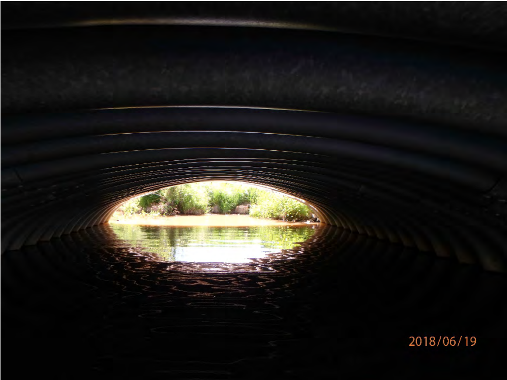
East through the Culvert
