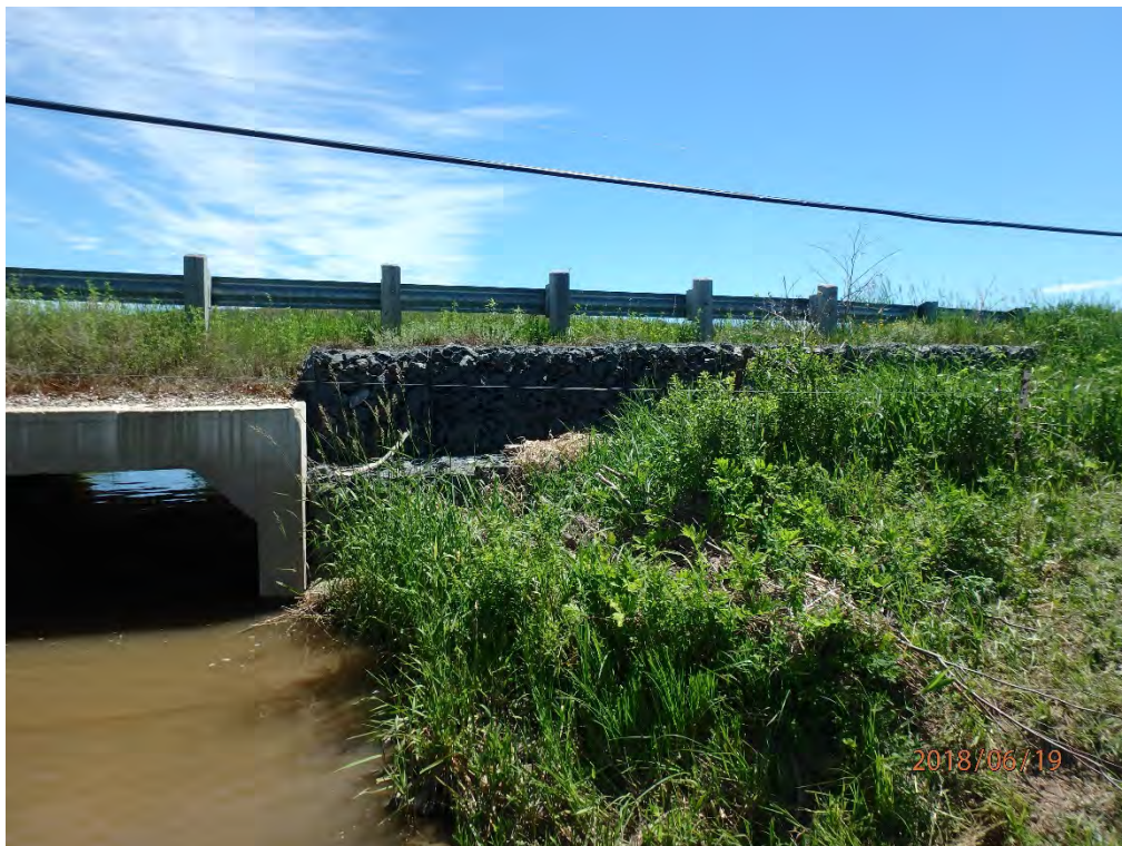
Gabions along west side of road
