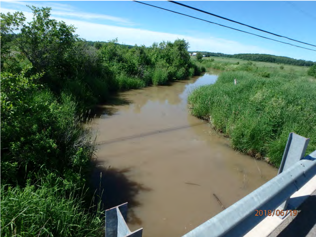
Downstream of bridge
