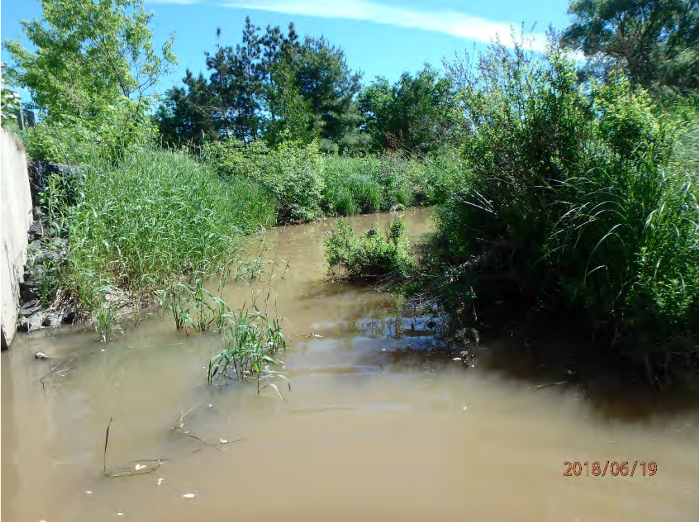
Downstream of Bridge
