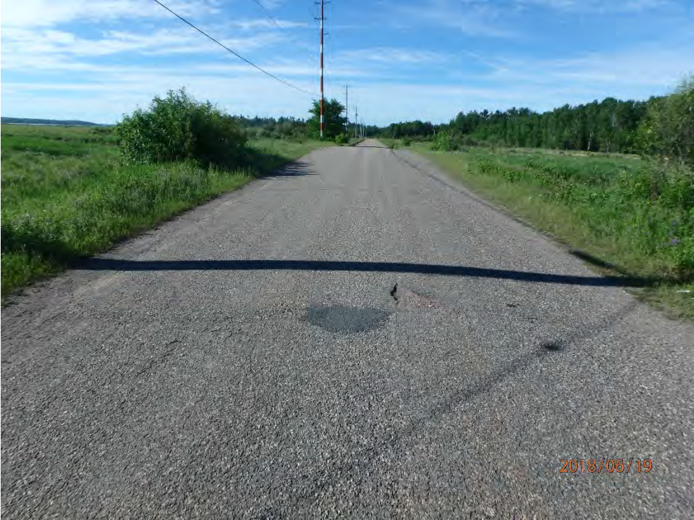
South across the culvert
