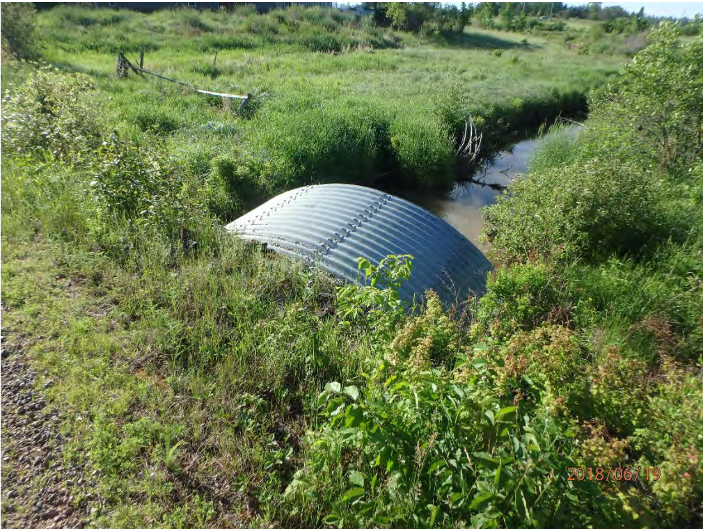
Downstream of culvert. Page wire fence across the creek.
