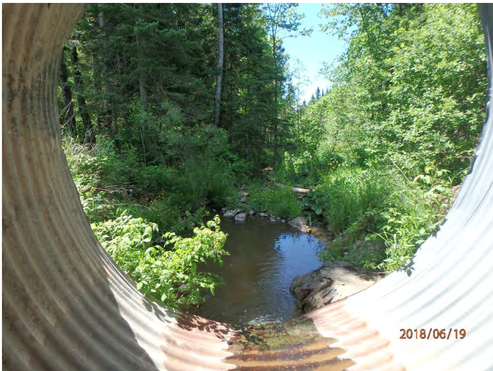
Outlet of culvert, looking south downstream.
