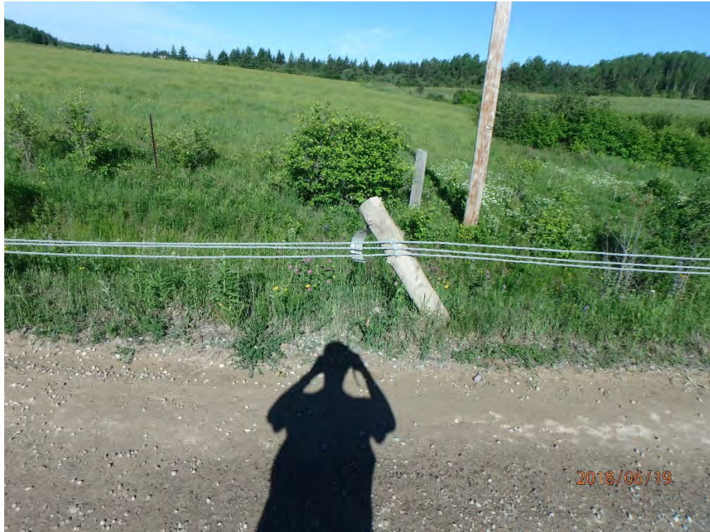
Broken post and slack in the steel guild cables
