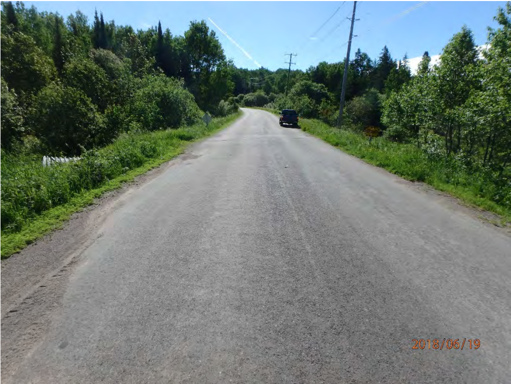
East across culvert
