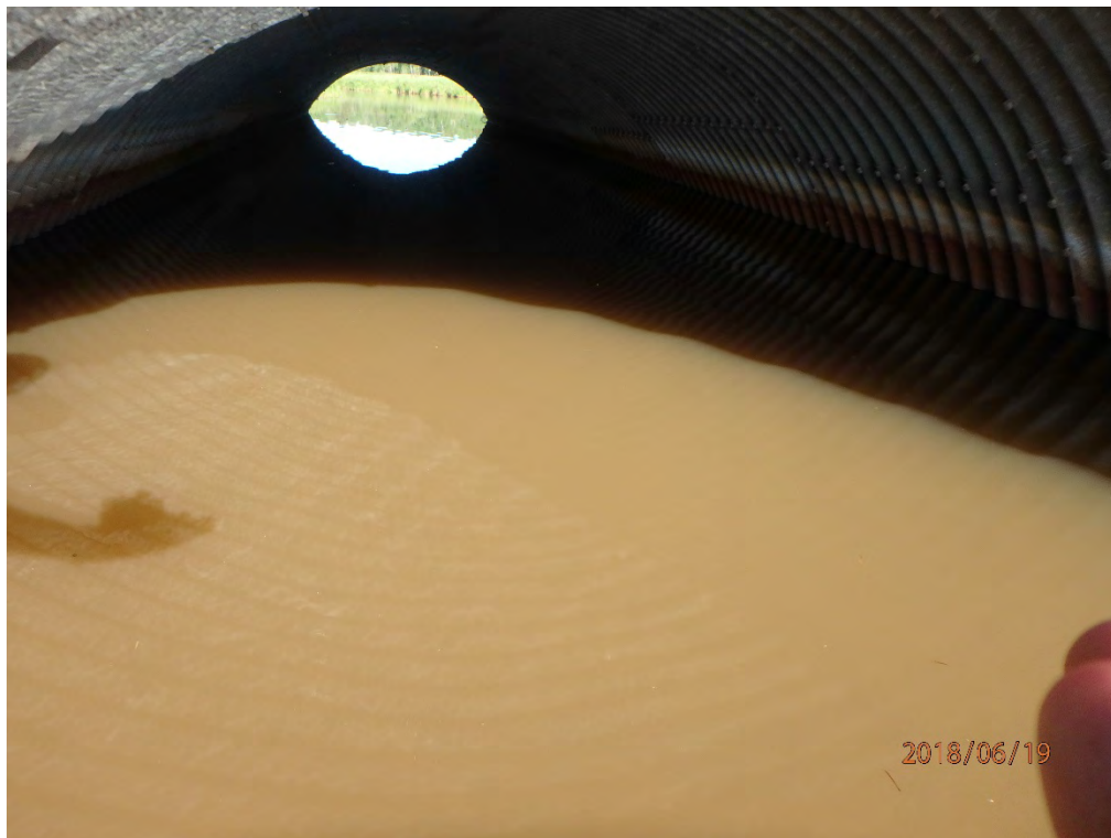
Looking upstream though the culvert
