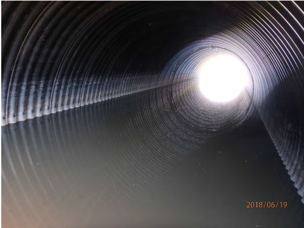
Looking north through the culvert.
