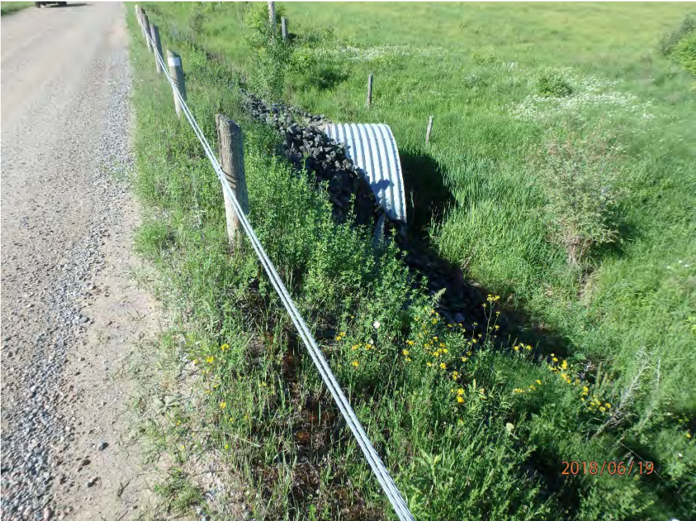
West end of the culvert, inlet
