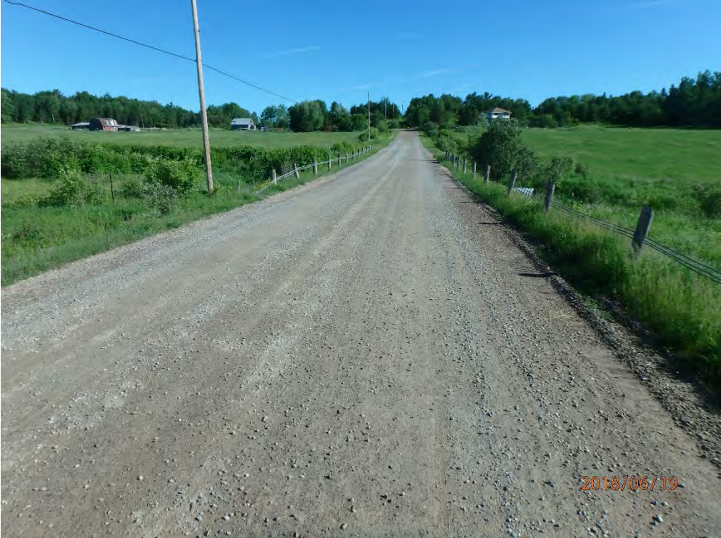
North across the culvert
