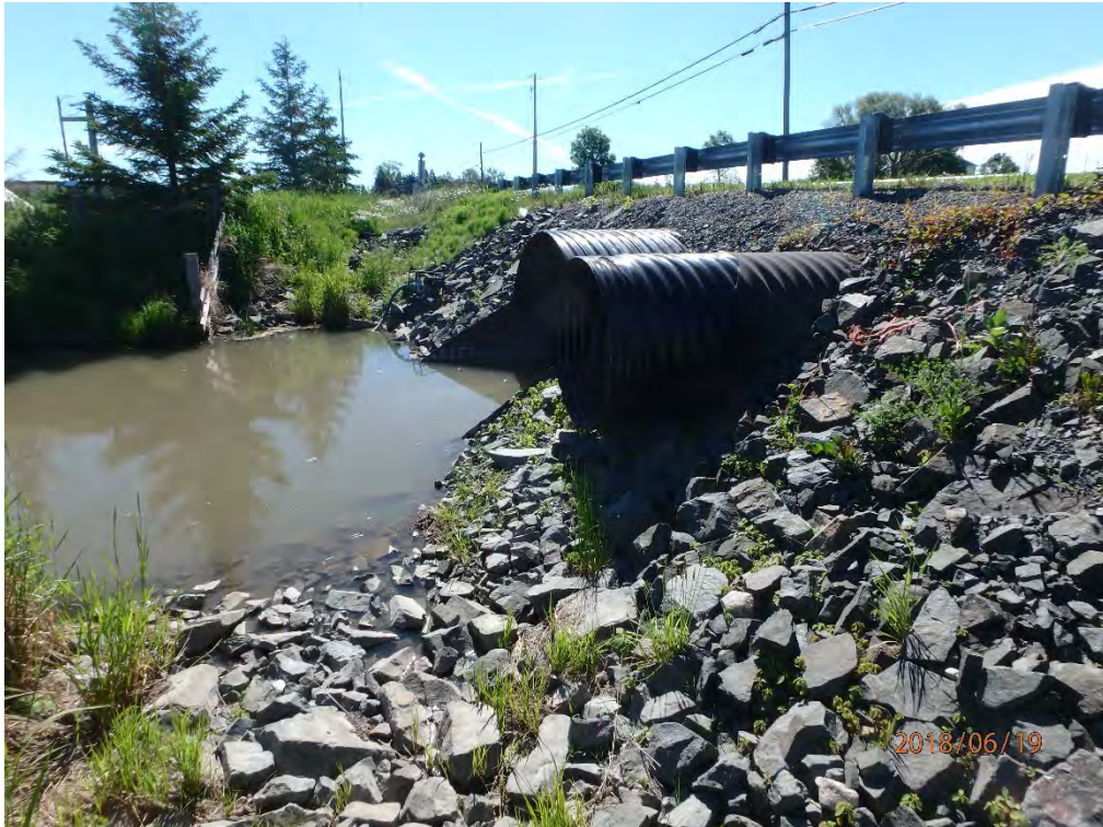
North side of Culvert, inlet. Banks protected by rock
