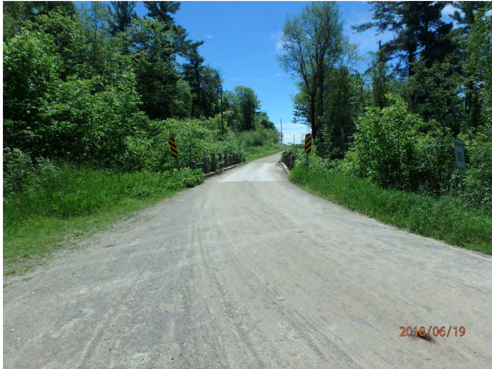
South across bridge
