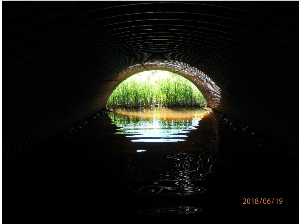
East through the culvert
