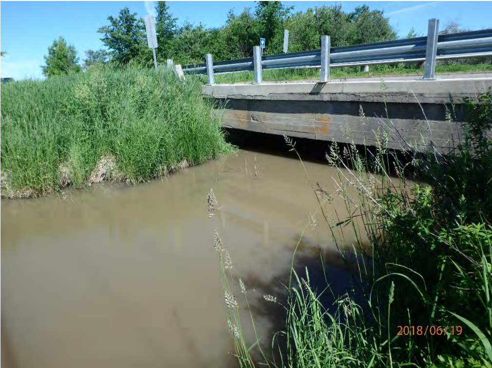
South Elevation of bridge
