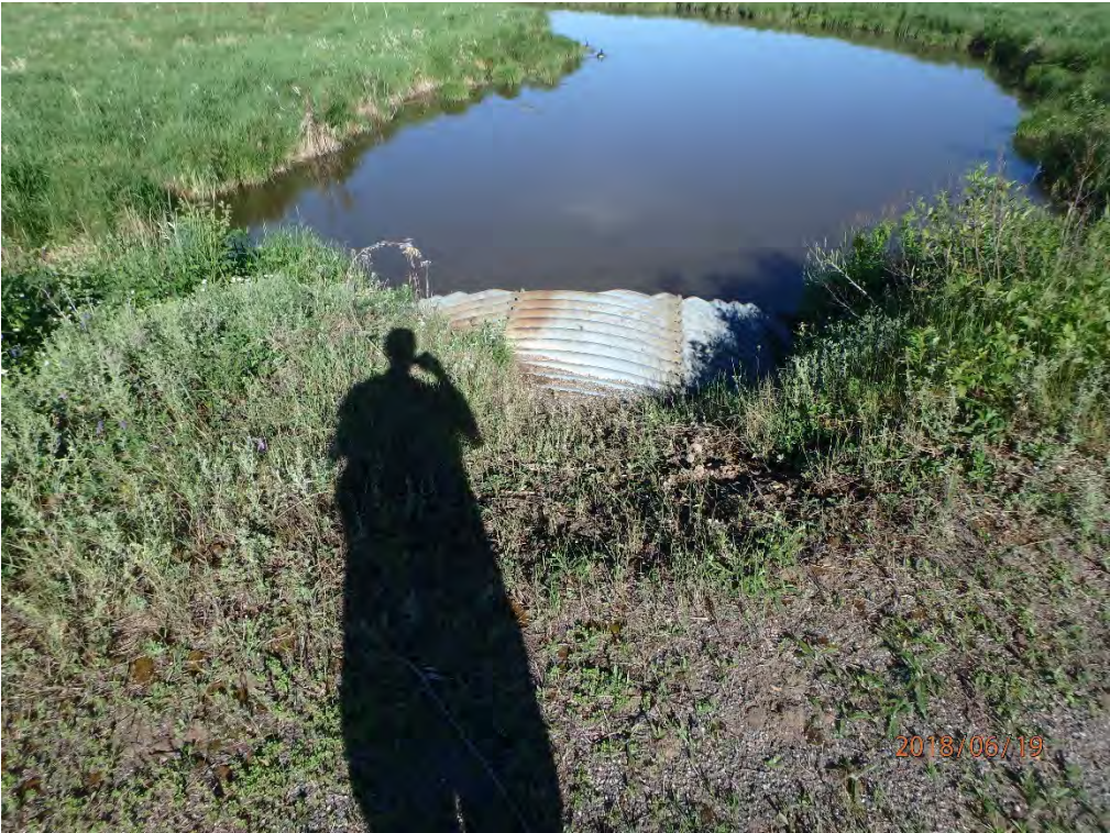
Looking west upstream of culvert
