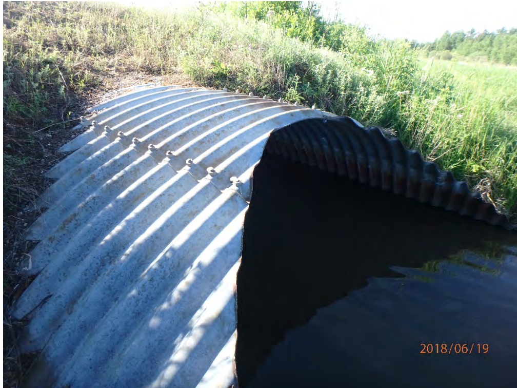
West elevation of culvert
