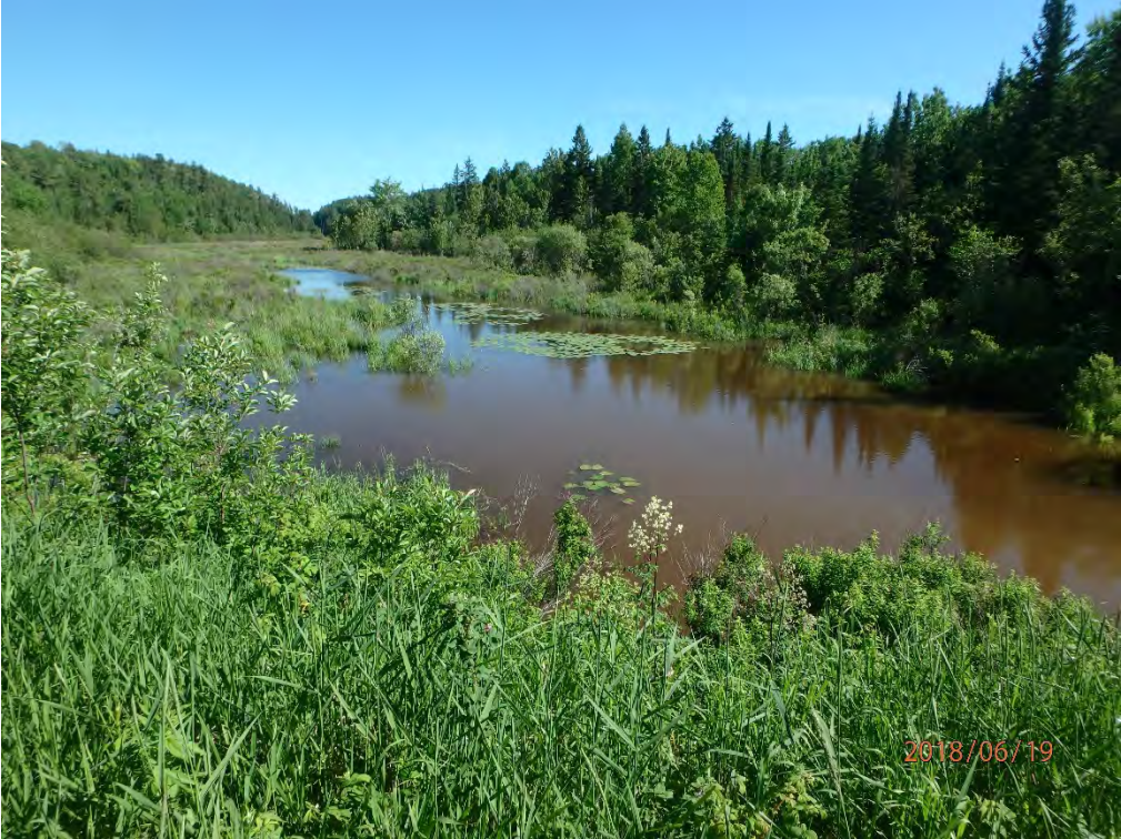
North upstream of culvert
