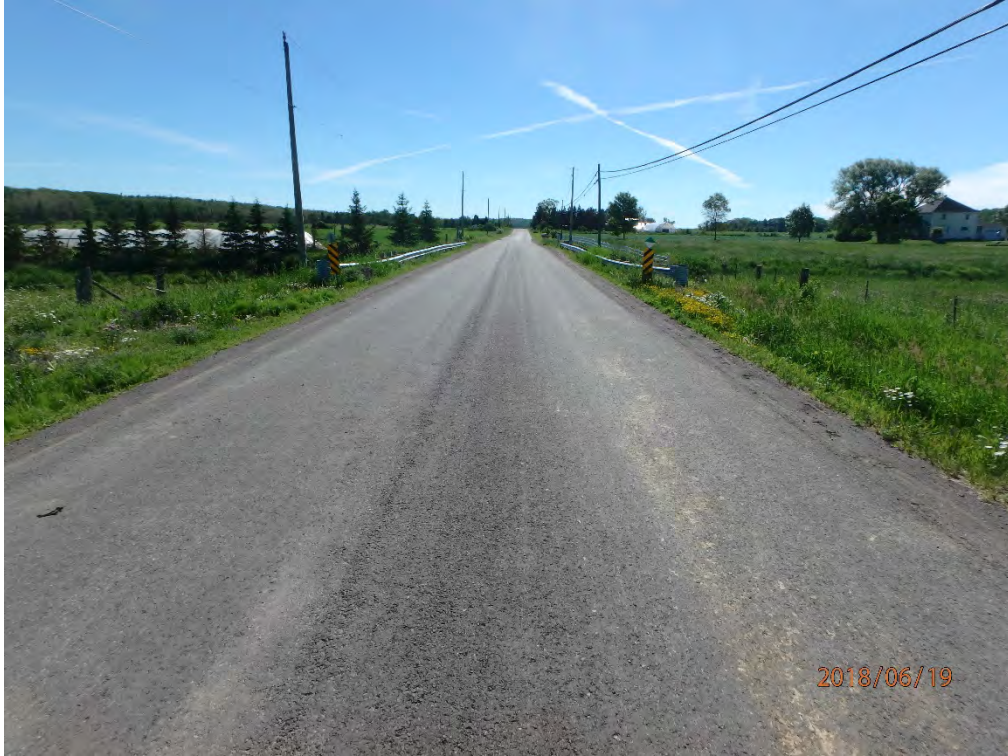
East Across culvert
