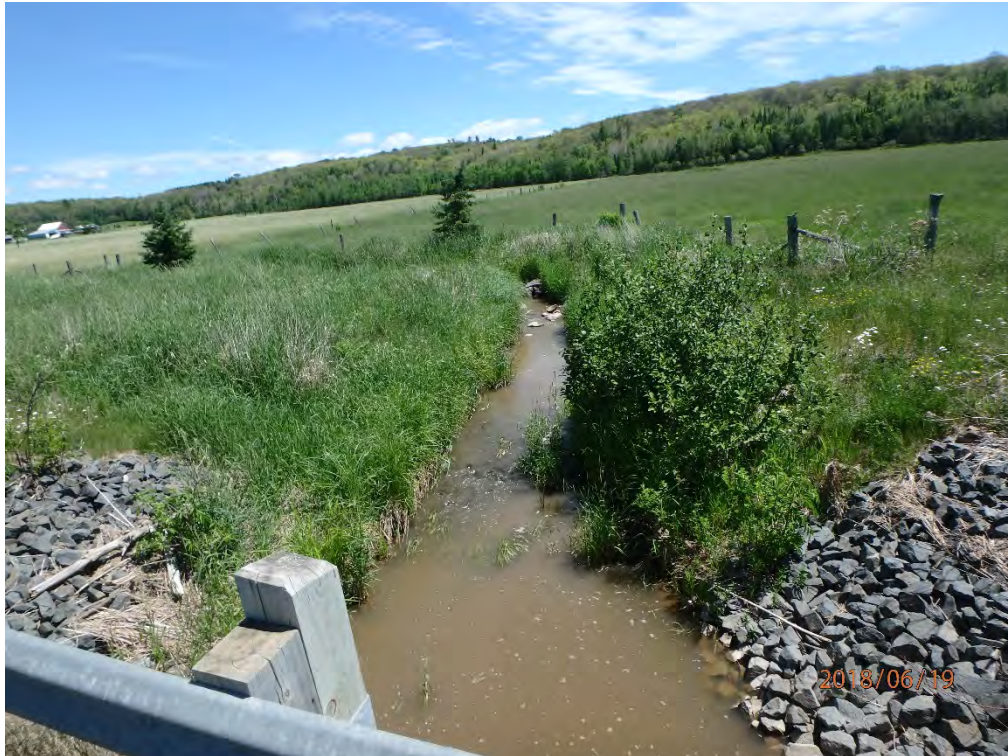
Looking downstream of the structure
