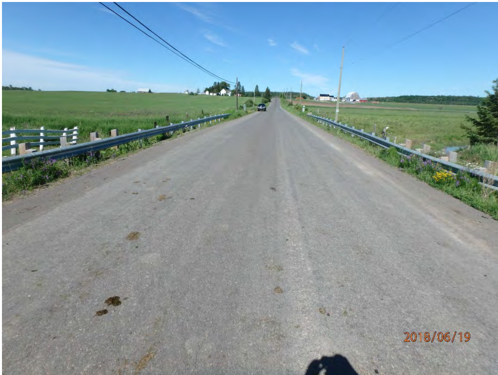
West across culvert
