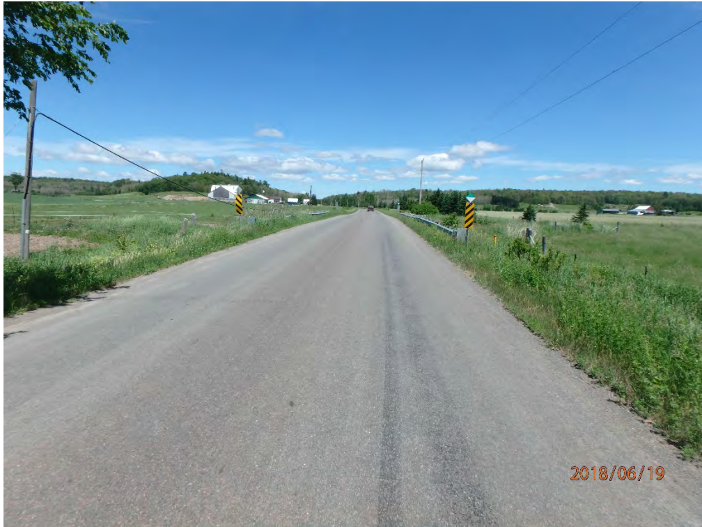
North across length of bridge
